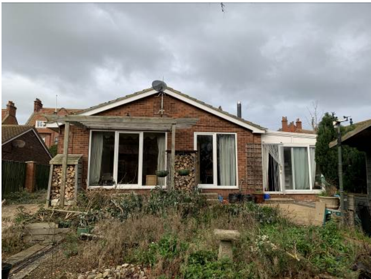
Photograph showing rear elevation of Elmford
