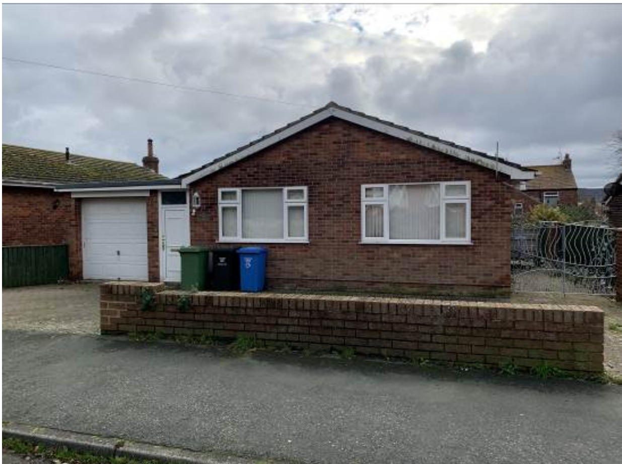
Photograph showing front elevation of Elmford
