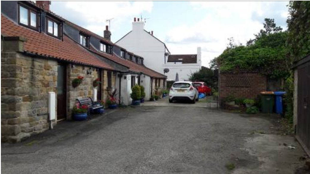
View of cottages form rear courtyard area
