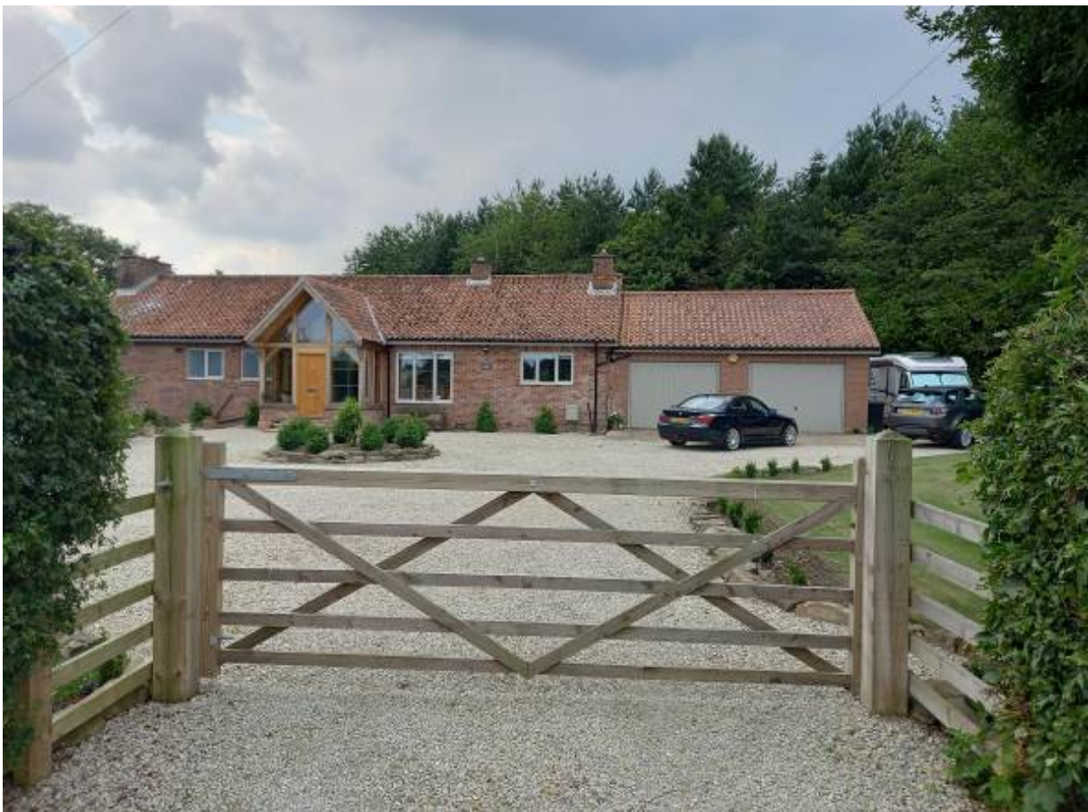
Photograph showing front elevation of 113 Hackness Road
