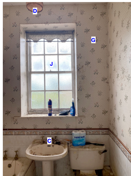
fig 9: Strip out existing fittings, fixtures and finishes
