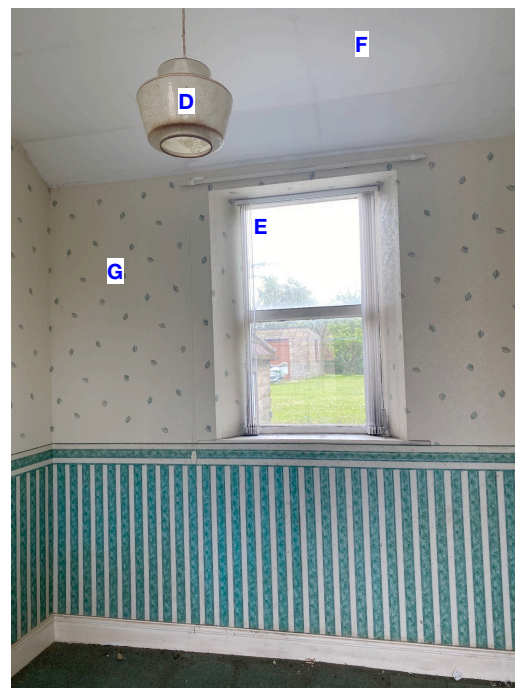
fig 7: replace upvc windows to rear elevation with timber double glazed sash windows
