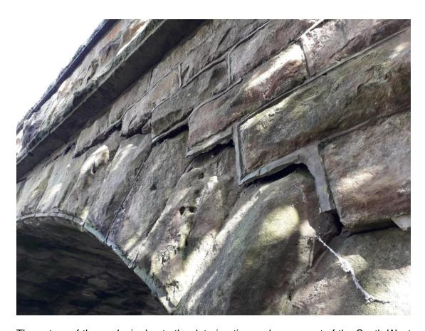
The nature of the works is due to the deterioration and movement of the South-West spandrel wall and South-East wing wall. The works are to ensure the structure is suitably safe for public use and that no loss of character is endured if the stonework falls down.
