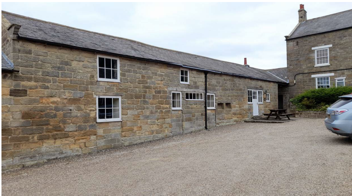
This is the internal east elevation of the courtyard.
