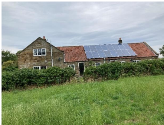
Fig 6. – South west elevation gable – Cottage 1 and Cottage 2.
