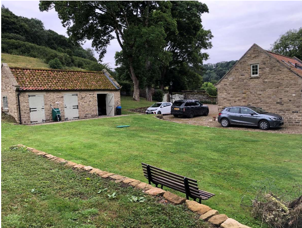
Photograph 1 General view looking to the Site Entrance showing existing Stable
