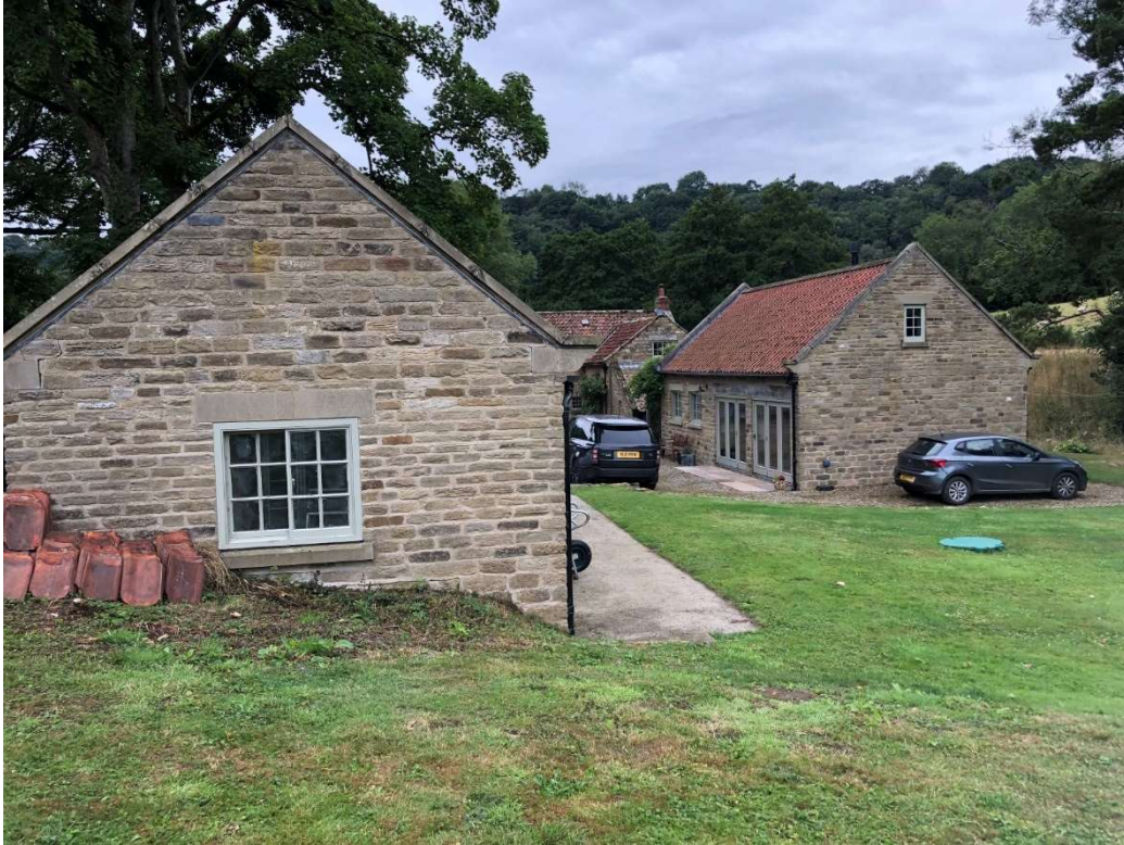
Photograph 3 View from the North showing the Gable of the Stable
