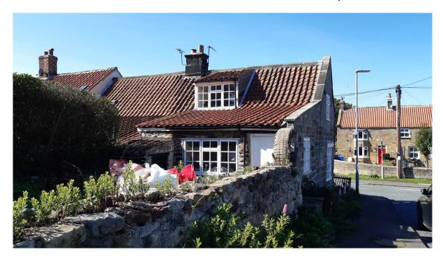
Side elevation of Laurel Cottage showing the cat slide pantile roof to the kitchen extension to be continued over the utility room and wet room extension and the dormer to be increased in depth
