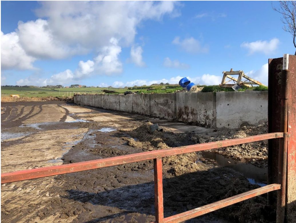
Fig 4. – Site of building proposed on opposite side of concrete panels.
