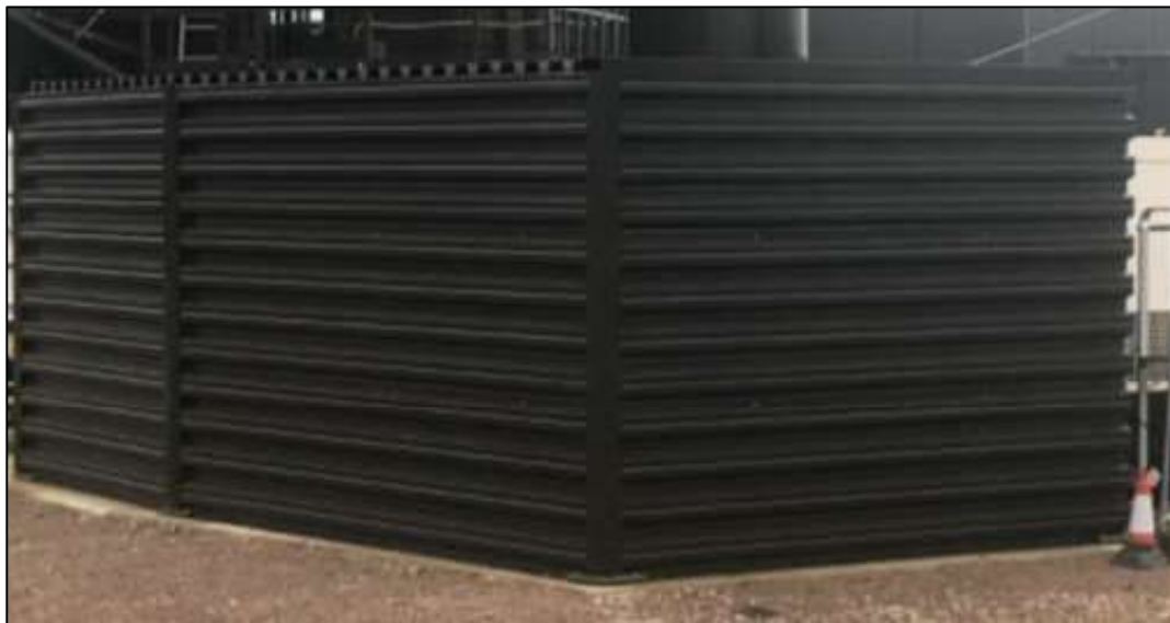
Image 5 – Winch enclosure, CWS-150 winch, steel frame and set-up for the emergency rescue winch
