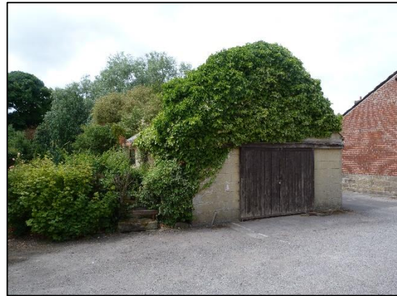
Photo 14: East gable wall.
