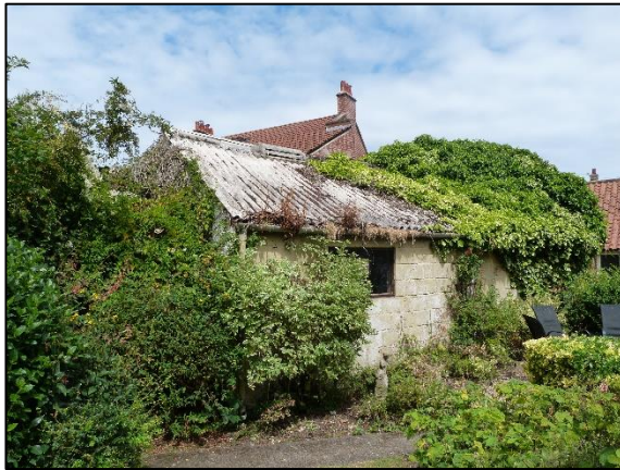
Photo 13: Building 1, south elevation.
