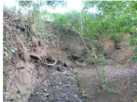
Photo 4: Drain along boundary.
