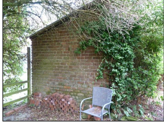
Photo 20: West elevation, Building 2.
