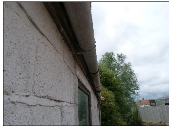
Photo 16: Well-sealed walltop.
