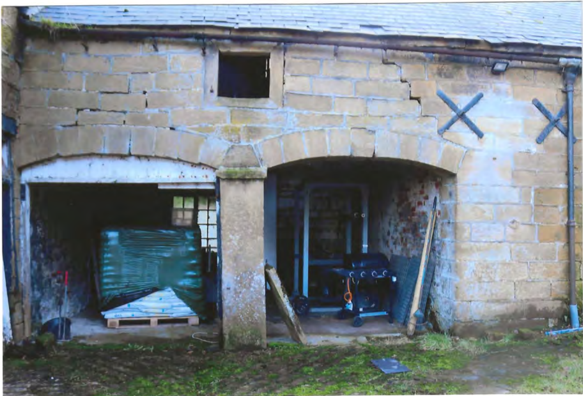
8. STONE ARCHES TO UNIT 2
