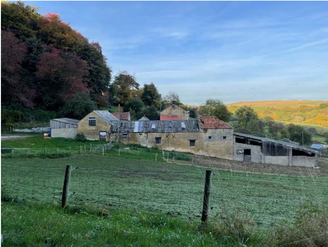
Elevation B showing stone outbuildings centrally flanked by relatively modern concrete block walled buildings to west and east that it is proposed are demolished
