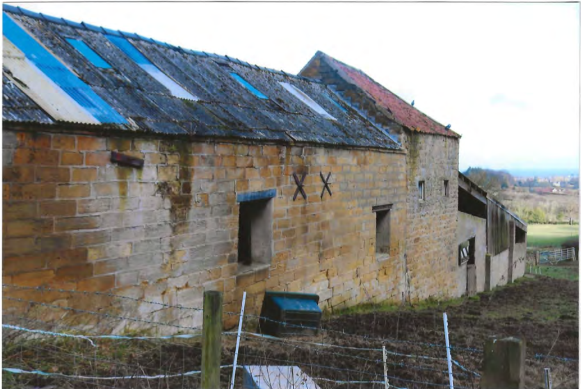
6. CLOSER VIEW ALONG SOUTH WALLS
