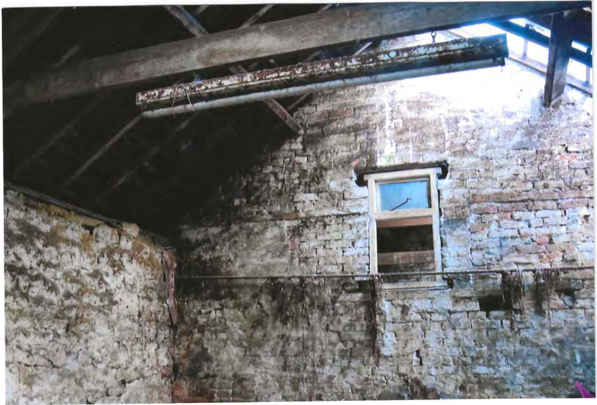
15. INTERNAL CROSS WALL - UNIT 2
