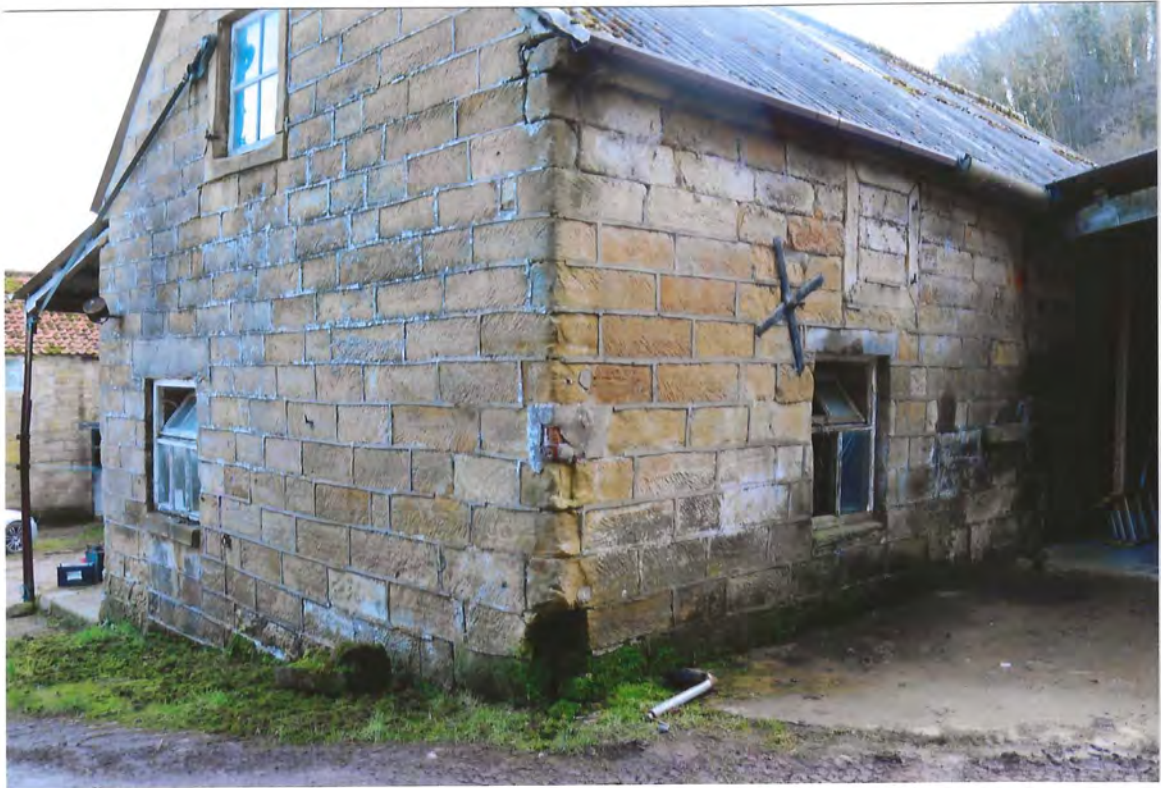
9. GABUE, REAR WALLS TO UNIT 1.
