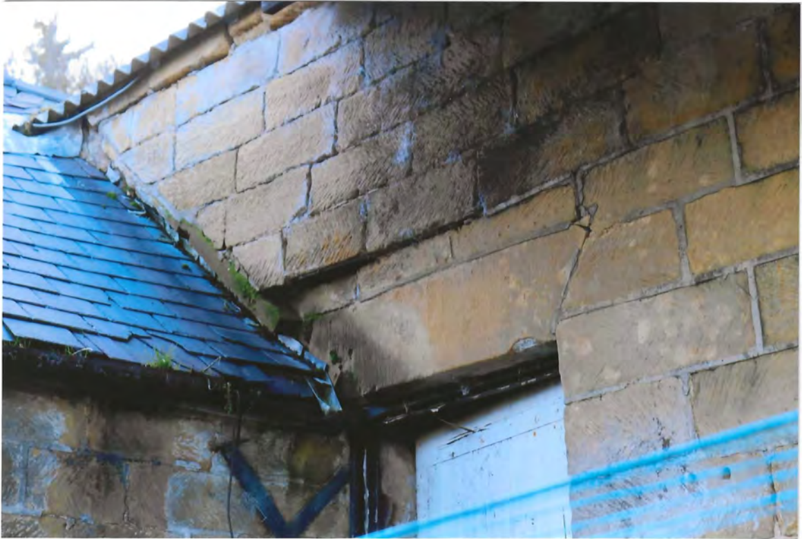
11. HORIZONTAL MOVEMENT - UNIT 1
