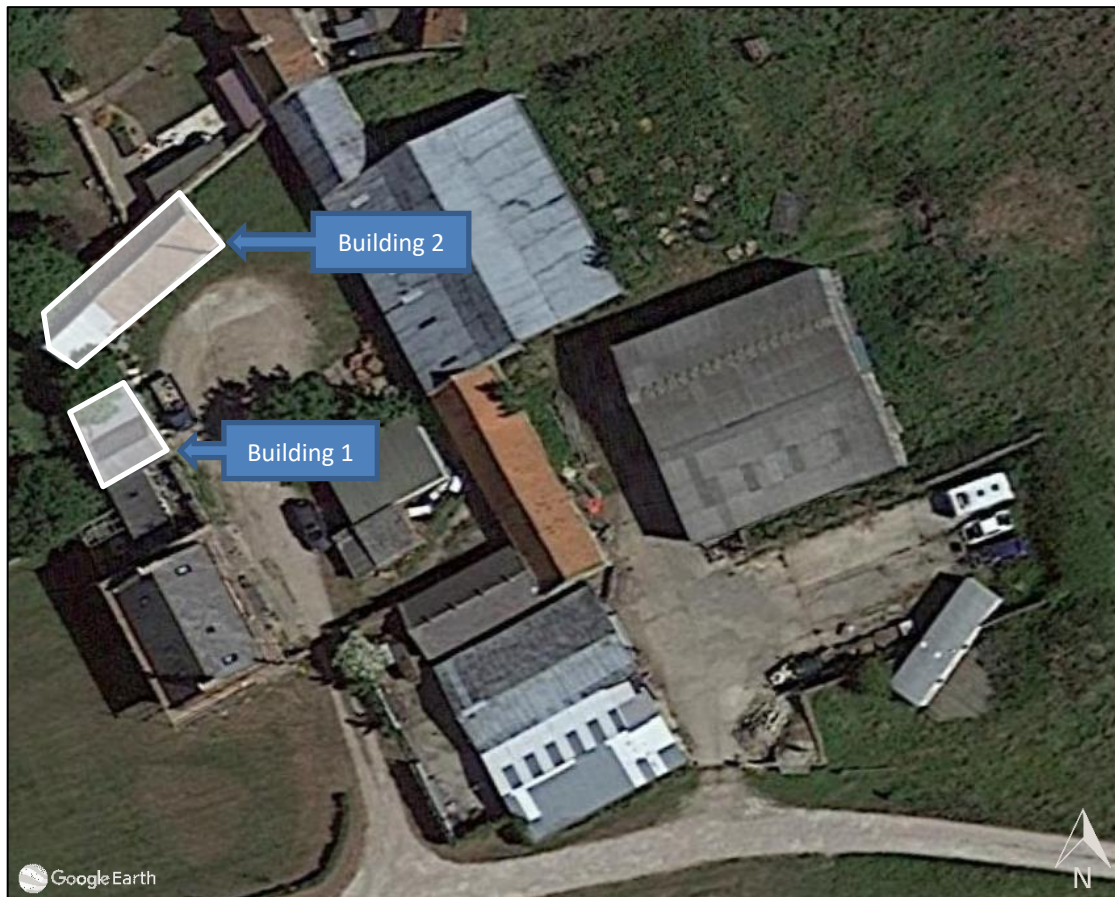
Figure 2: Location of surveyed buildings at Low Laithes Farm. (Google Earth 2023.)
