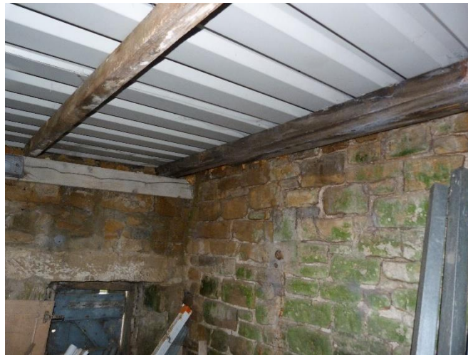
Photo 6: Internal view of flat roofed section.
