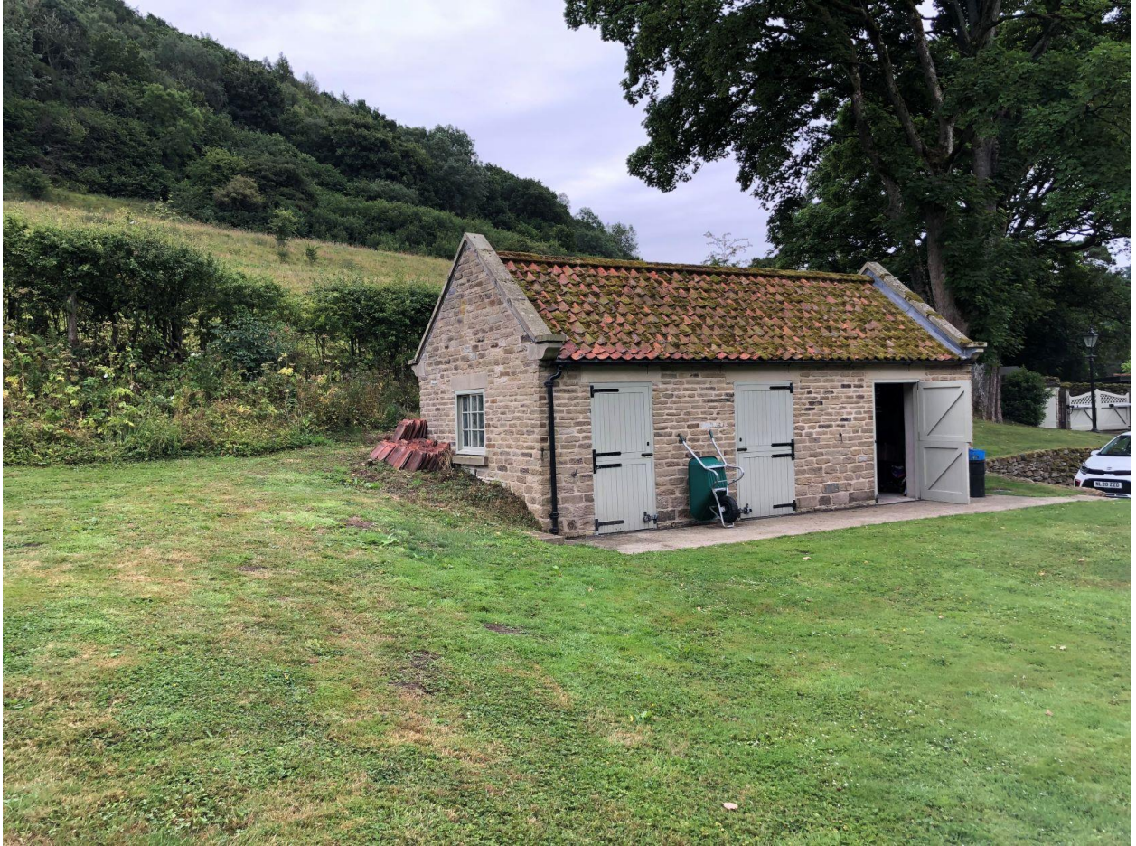
Photo 2 Stable viewed from the West
