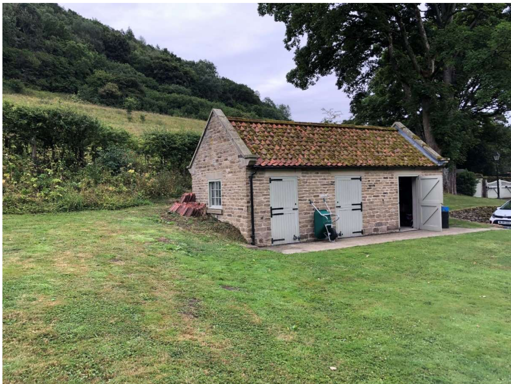
Photograph 2 Existing Stable viewed from the West
