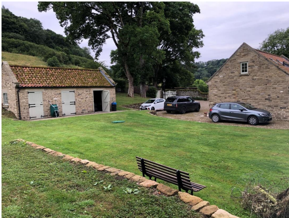
Photo 1 General View looking to the Site Entrance showing existing Stable
