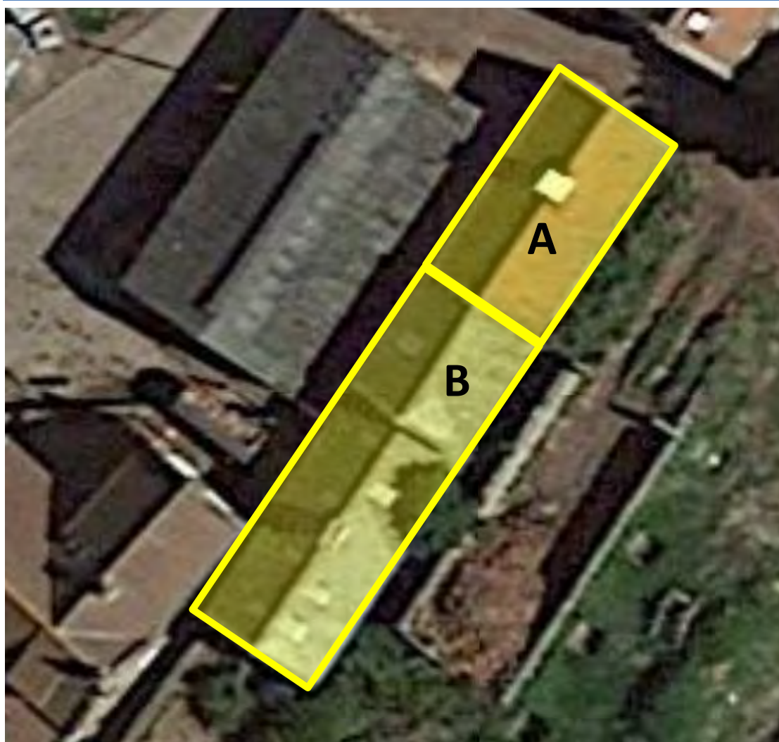
Figure 4: Aerial view of the surveyed building.
