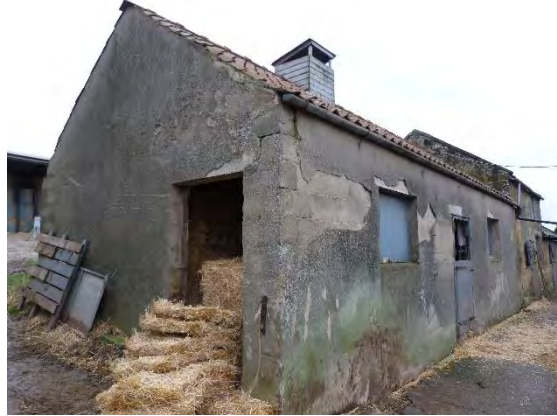
Photo 1: View of the building. South aspect.
