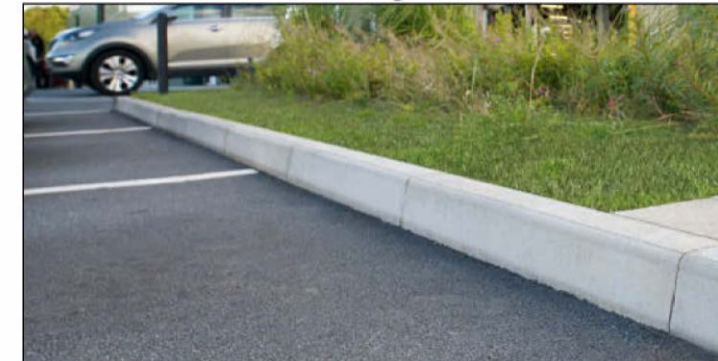
Kerb and Tarmac.
