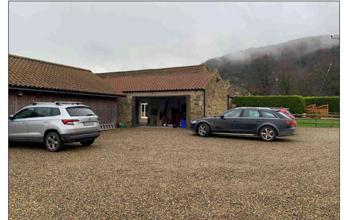
Garage and rear of stables
