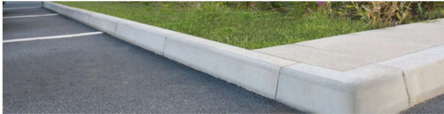
STANDARD CONCRETE KERB & BLACK TARMAC
