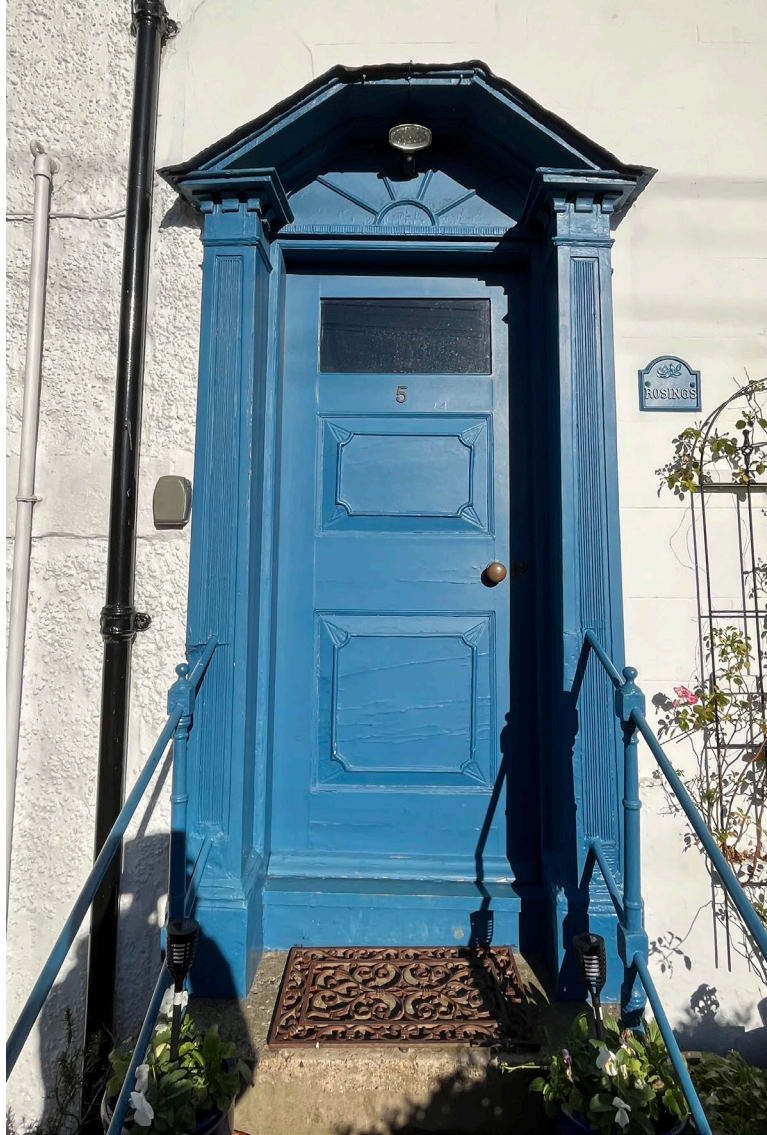
Photo 2 – detail of timber surround to No. 5 Bloomswell
