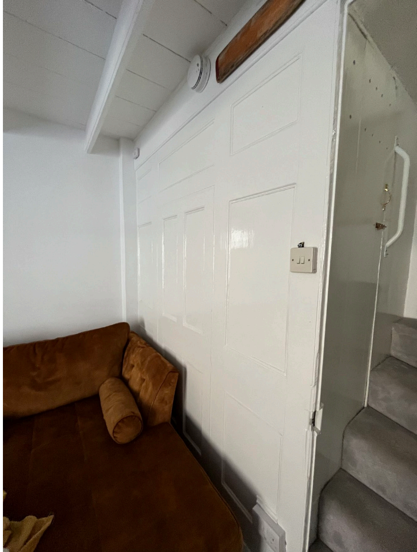
Photo 3 – detail of timber paneled partition in living room
