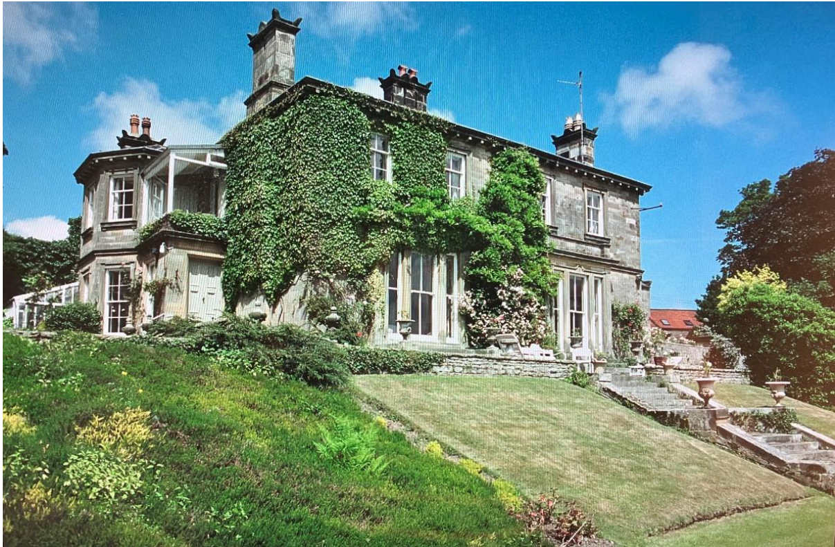
Fig. 9 – C21 photograph showing replacement lean-to and belvedere (now removed) from garden elevation.
