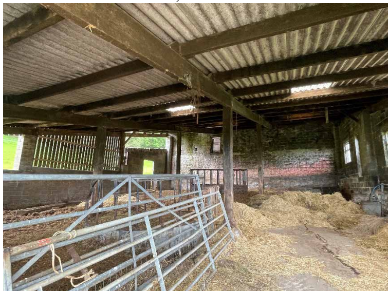
Plate 12 – Unit 3, internal roof structure.
