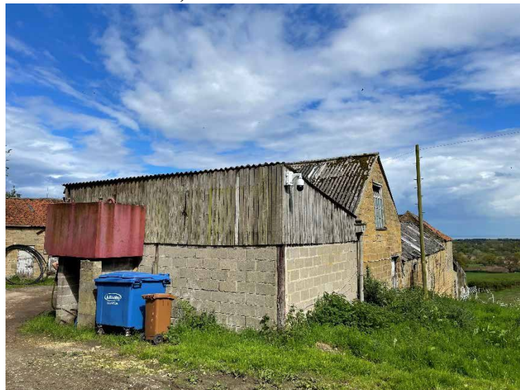
Plate 3 – Unit 1, northwest and southwest elevation
