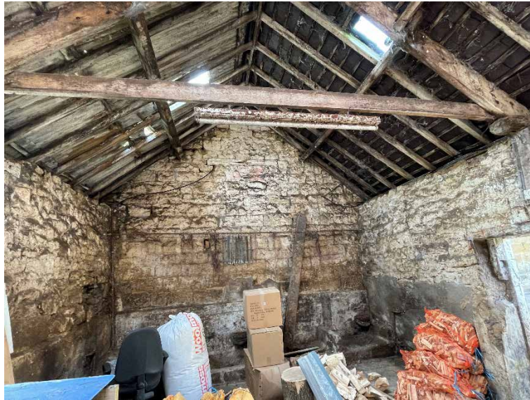
Plate 7 – Unit 2, internal roof structure.
