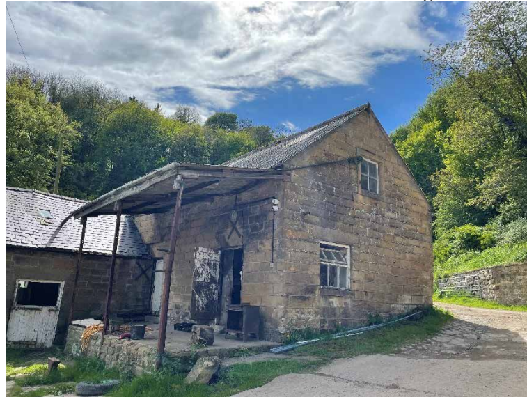
Plate 1 – Unit 1, east elevation and north gable.
