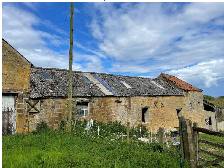
Plate 6 – Unit 2, southwest elevation.
