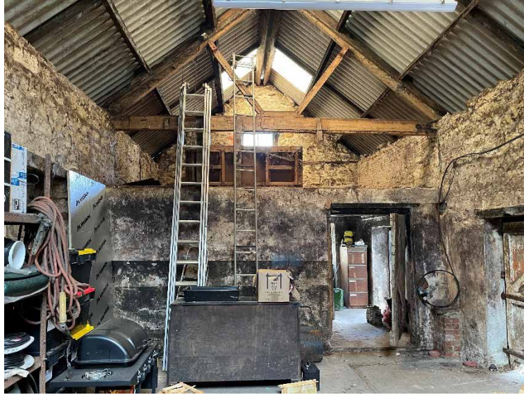
Plate 4 – Unit 1, internal roof structure.
