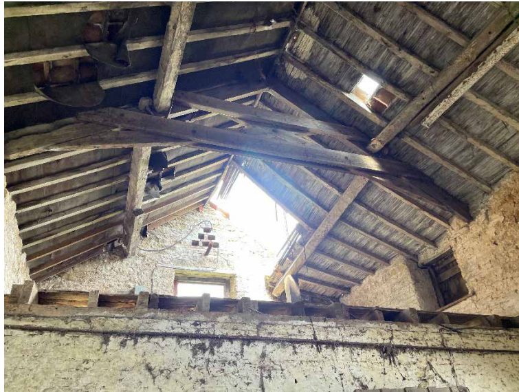
Plate 13 – Unit 3, internal roof structure.
