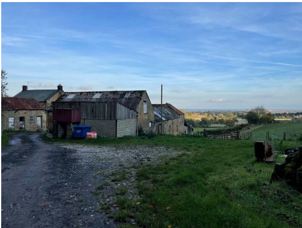
Elevations B & F with modern outbuilding in foreground (to be demolished leaving 3 car spaces for holiday guests)
