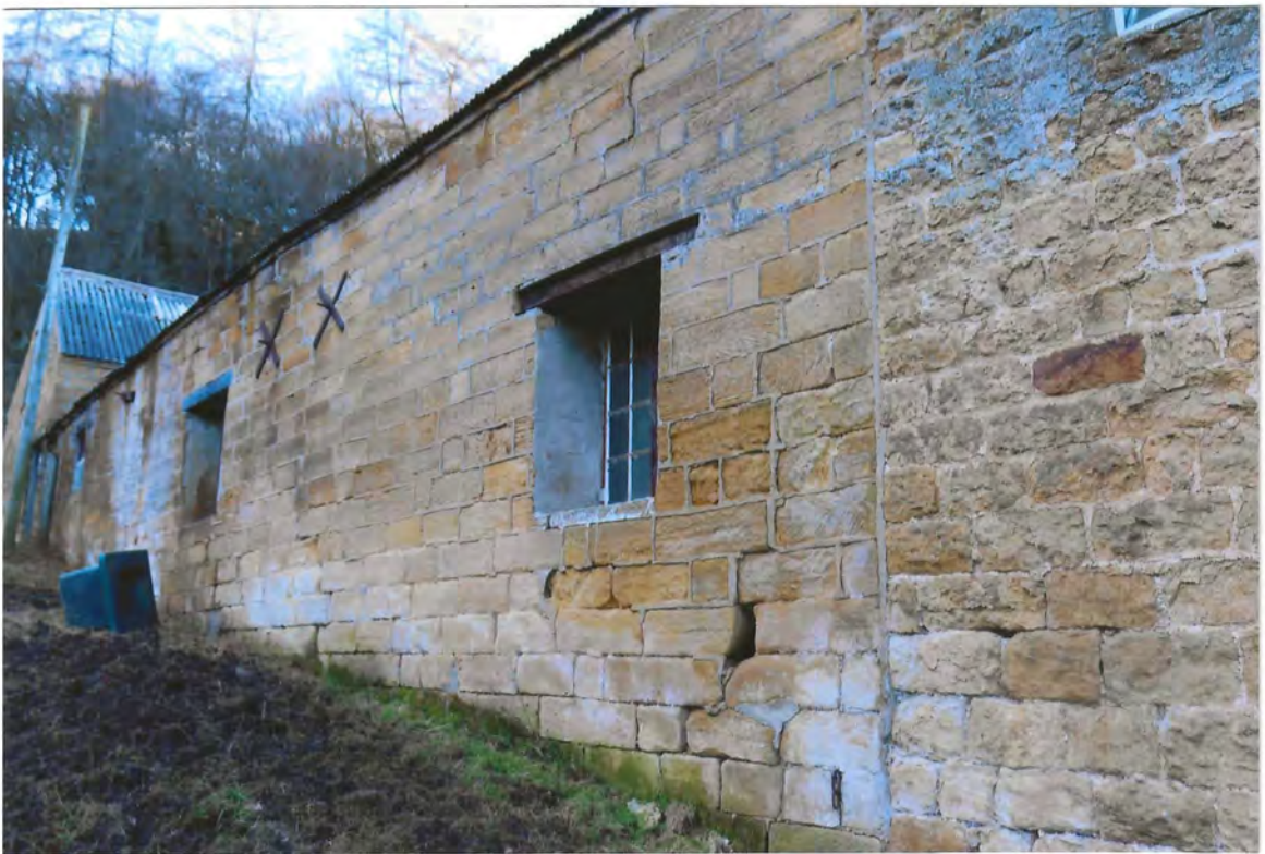
10. CLOSE UP VIEW ALONG SOUTH WALL
