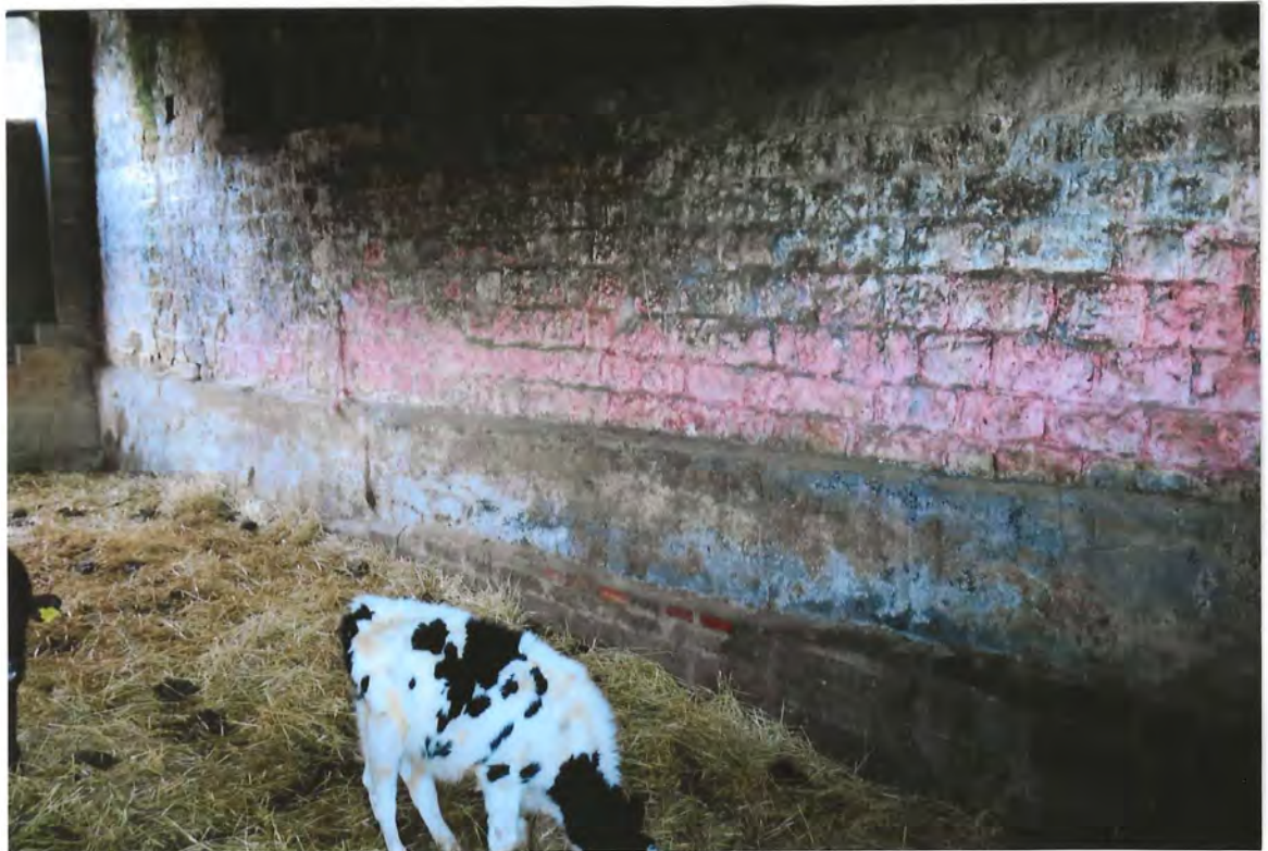
16. LOWER EXTERNAL WALL TO UNIT 3 EXISTING FORD YARD TO BE DEMOLISHED
