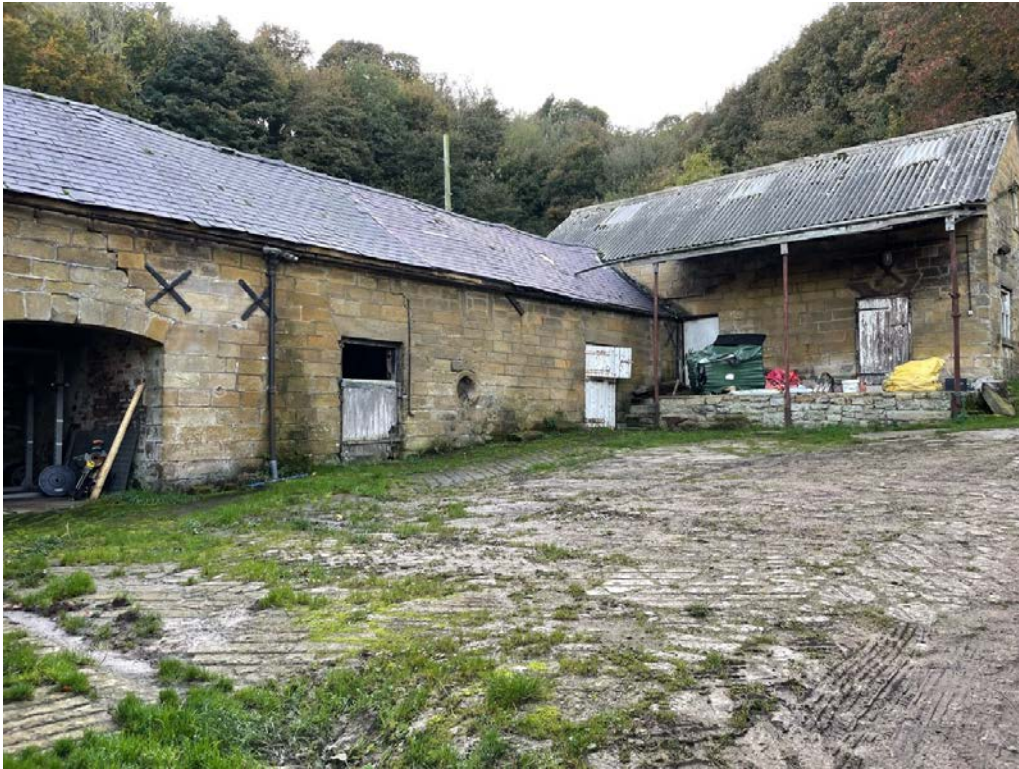
Elevations A & E again with courtyard area flanked by outbuildings
