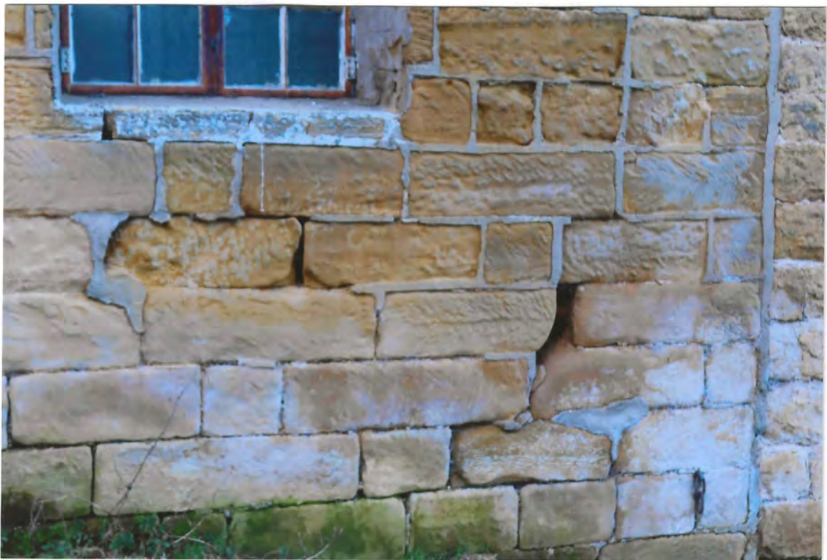
12 CLOSE UP OF SMALL SECTION ALONG SOUTH WALL
