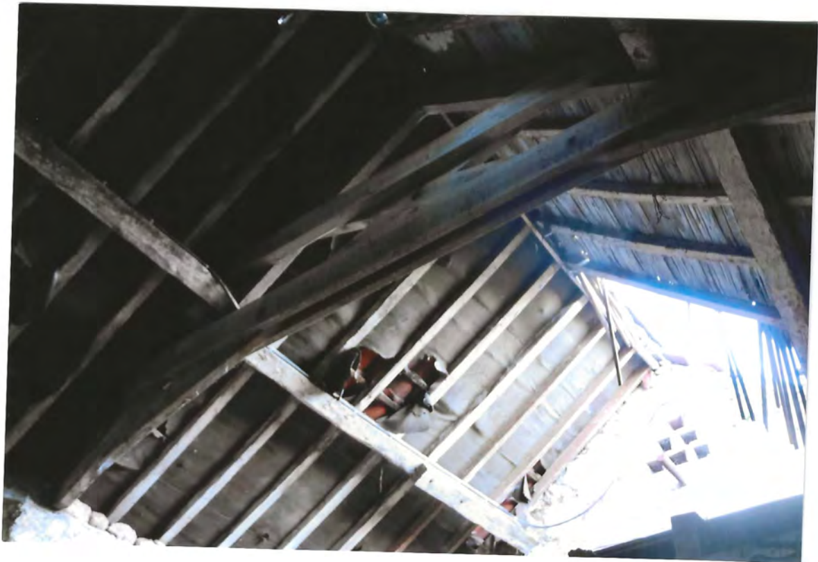
14. ROOF DETAIL . UNIT 3
