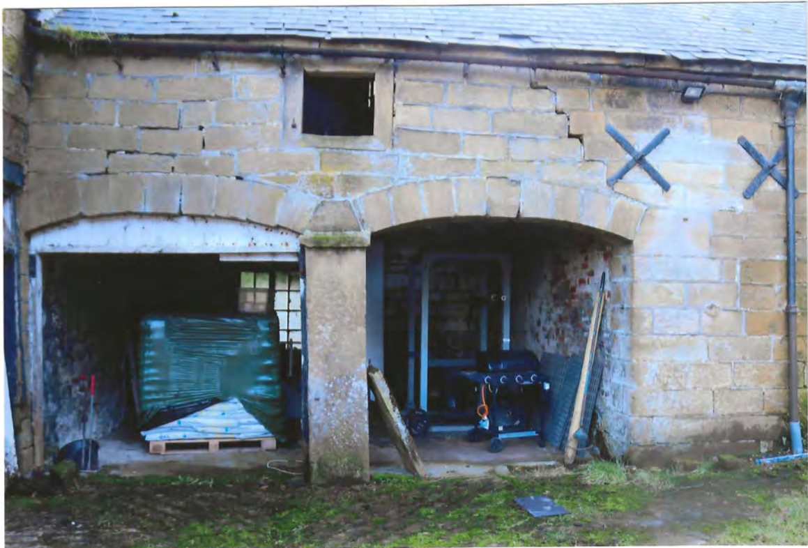
8. STONE ARCHES TO UNIT 2
