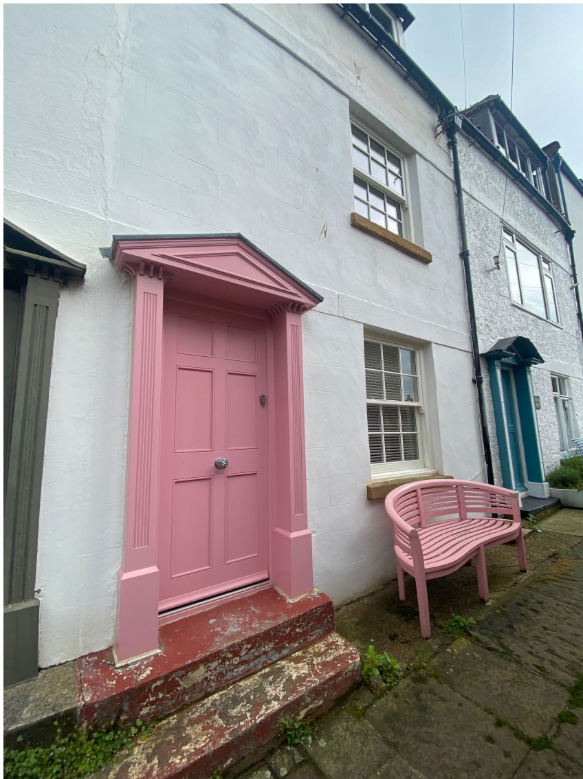
The unauthorised door and door surround at 3 Bloomswell
