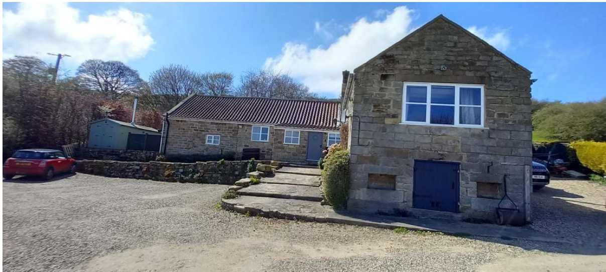
This shows the front elevation of Underhill Cottage and the attached outbuilding.
