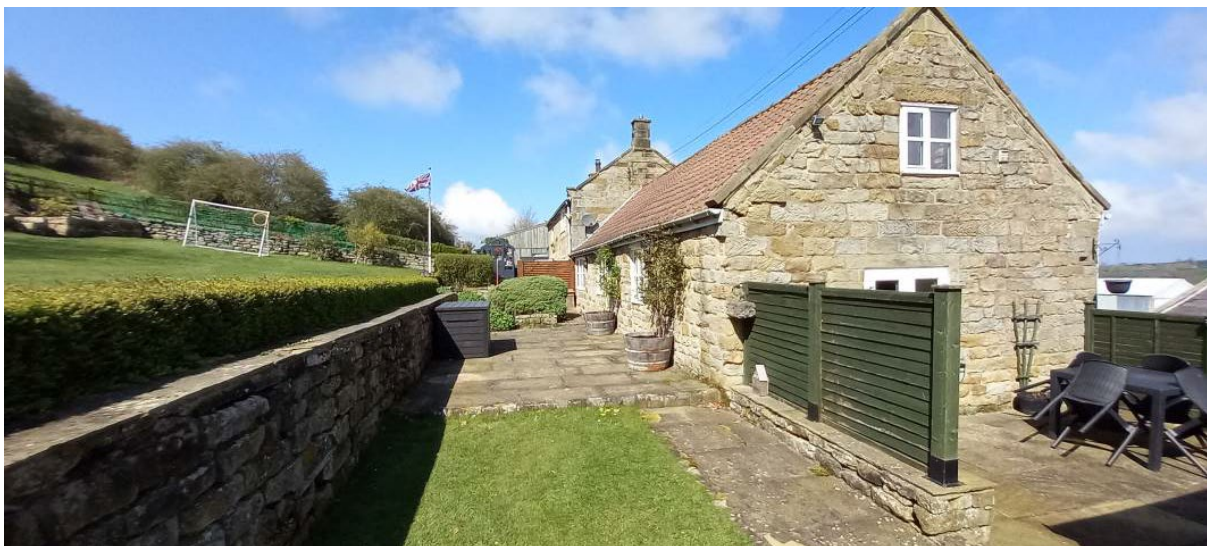
This shows the rear elevation of Underhill Cottage and the attached outbuilding.
