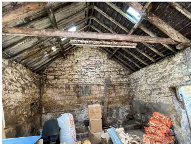
Plate 8 – Unit 2, internal roof structure.
