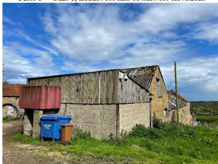
Plate 3 – Unit 1, northwest and southwest elevation.
