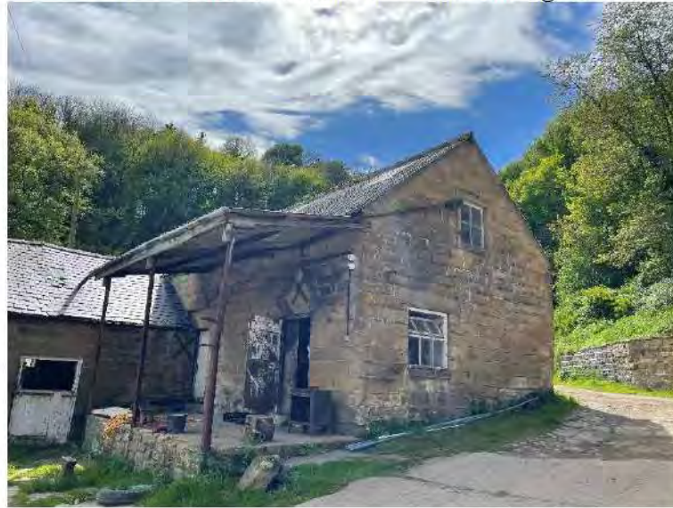
Plate 1 – Unit 1, east elevation and north gable.
