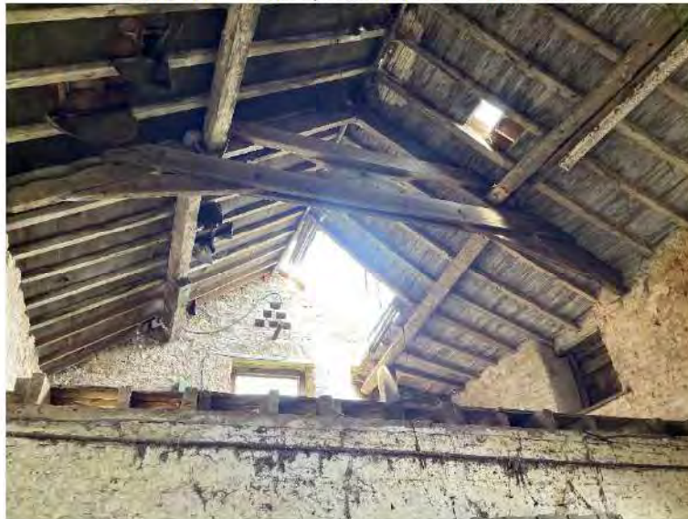
Plate 14 – Unit 3, internal roof structure.
