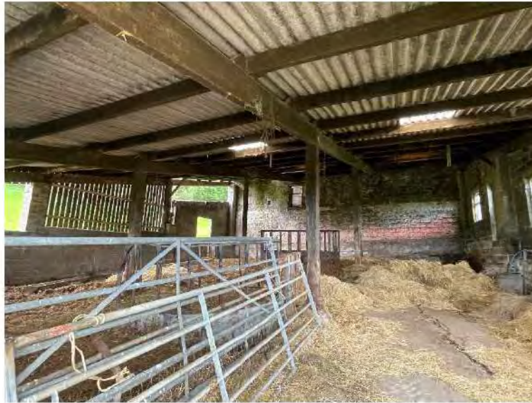
Plate 13 – Unit 3, internal roof structure.
