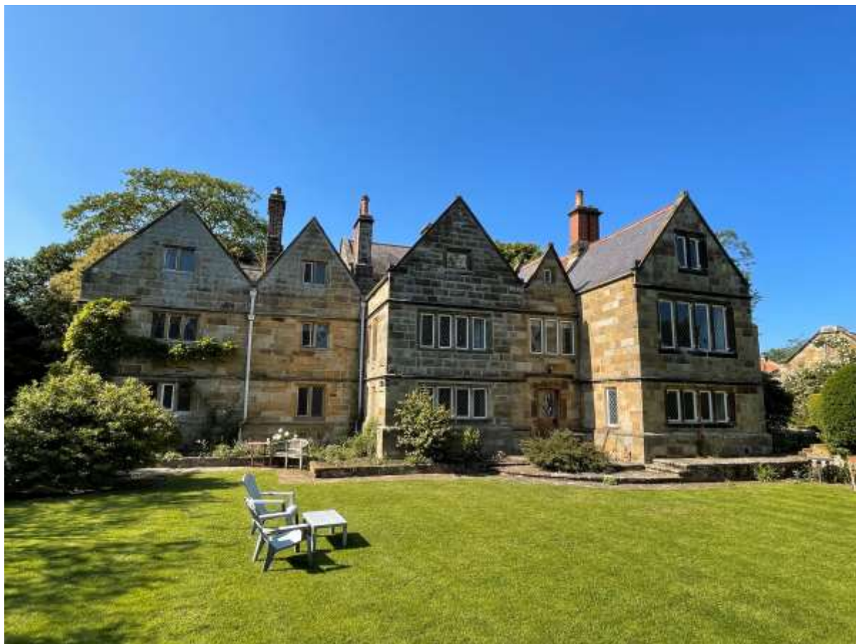
Figure 20 - Southeast facing elevation of 'Original House', 1835 addition, link building, 1844 incorporated building and south roof slope of Storeyed porch. Southern roof to be utilised for Solar PV.
