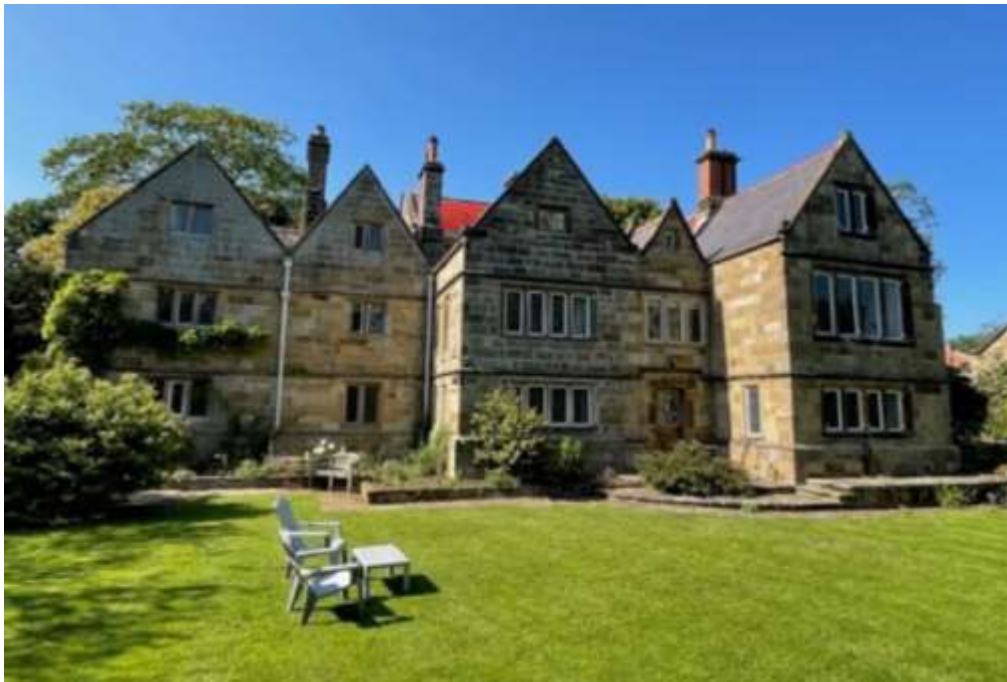
Figure 10 - Southeast elevation showing effect of PV array (RED) to south facing roof and minimal impact on heritage building
