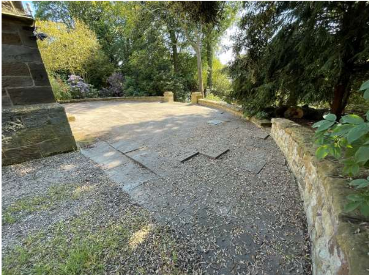
Figure 17 - Existing terrace to South West Elevation. Existing concrete pavers shown. Paving to be removed and replaced with yorkstone flagstones or bonded gravel.
