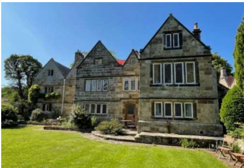
Figure 11 - Southeast elevation showing effect of PV array (RED) to south facing roof and minimal impact on heritage building
