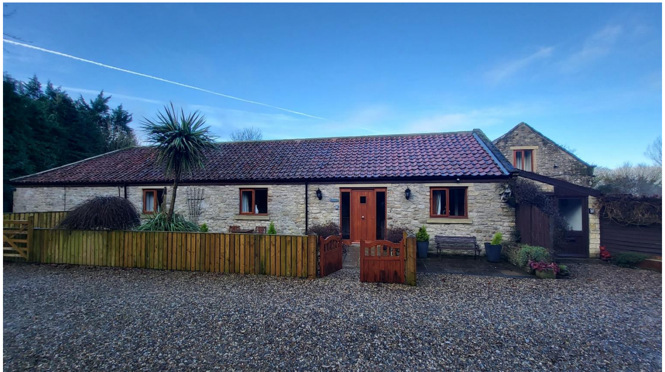
Image 4: eastern elevation of single storey units
