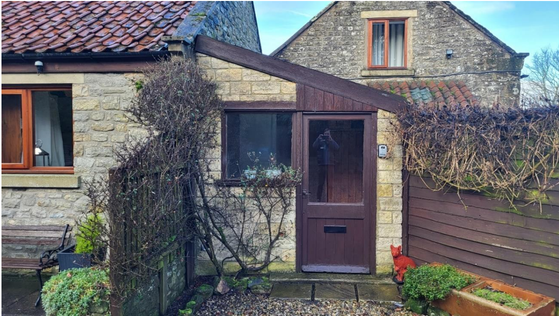
Image 1: existing extension to be demolished:
