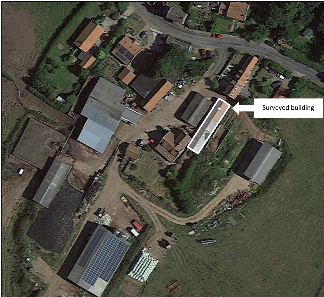
Figure 2: Aerial view of surveyed building at High Farm. (Google Earth 2023.)
