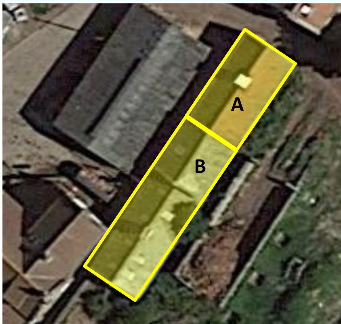
Figure 4: Aerial view of the surveyed building.
