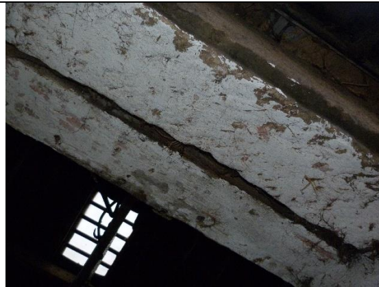
Figure 17: Gap in door lintel.
