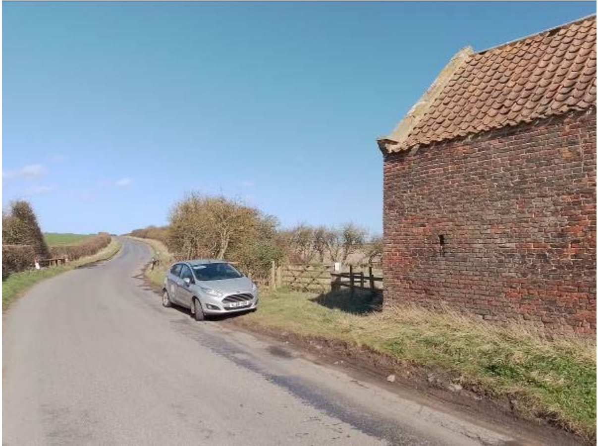
Photo showing Red Barn (Listed Grade II) and gate into field where caravan would be located
