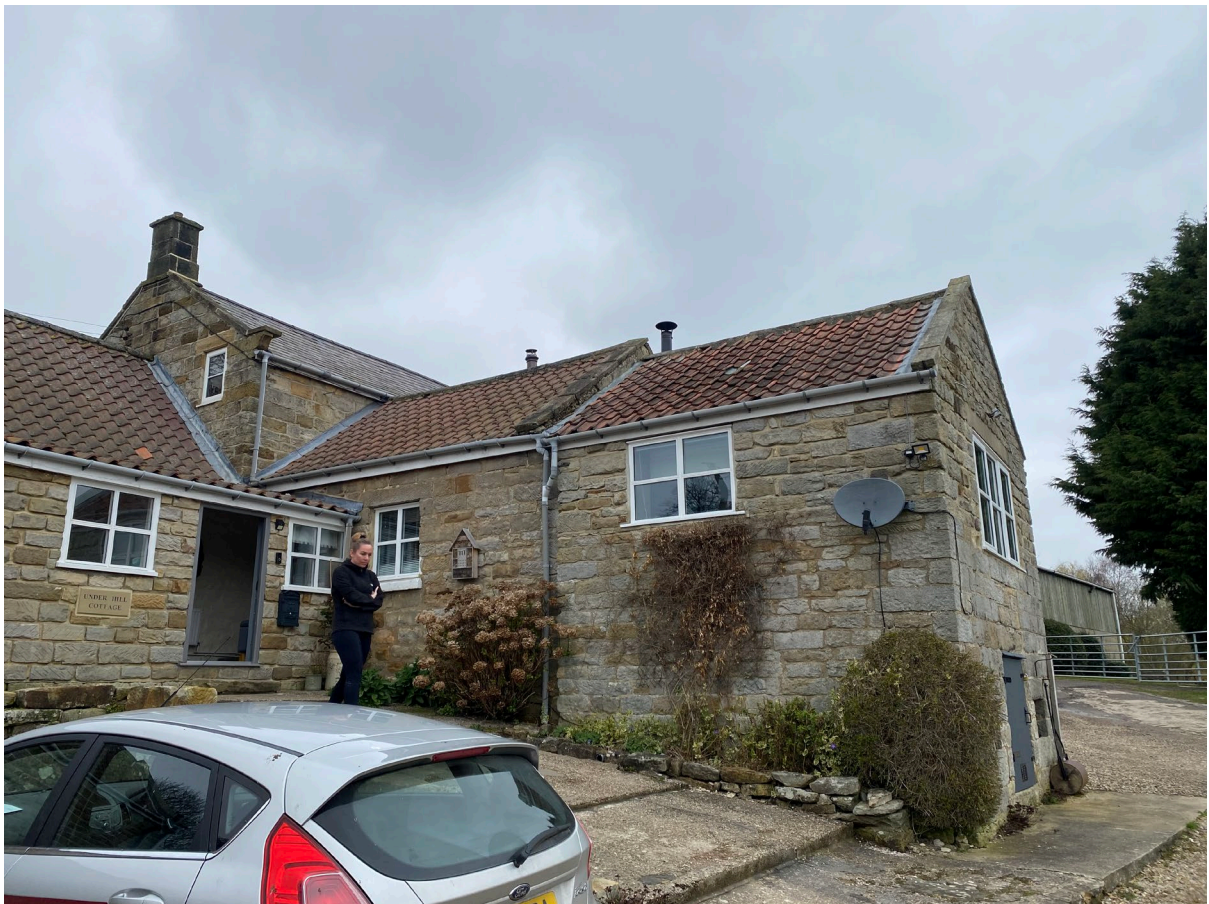
This photo shows the south elevation rear outshot that the application proposes to raise the height of.
