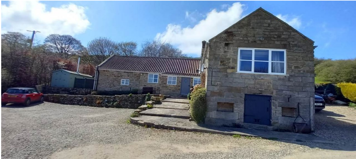
This photo shows the east elevation of the dwelling, as existing.
