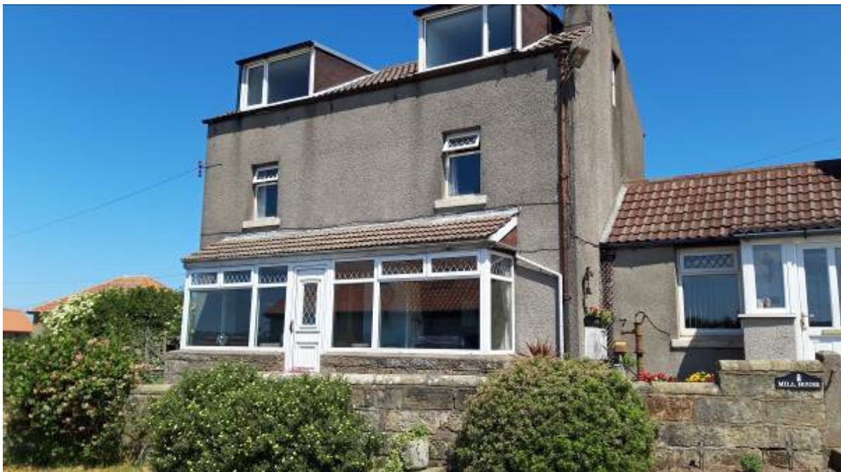
Photograph showing front elevation of Mill House, Low Hawkser
