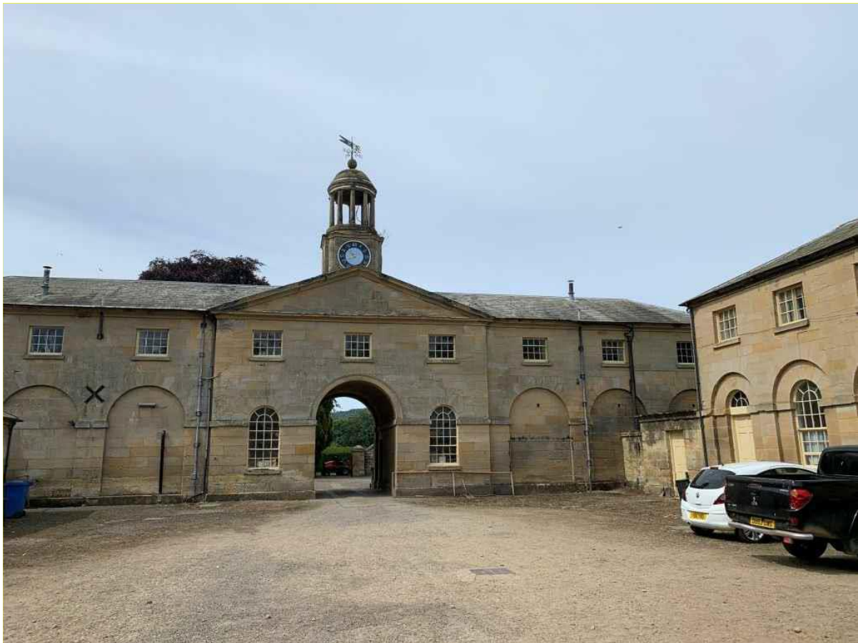
Figure 1: Images to show the Grade II Listed Building, the existing telecommunication site for the proposed upgrades.
