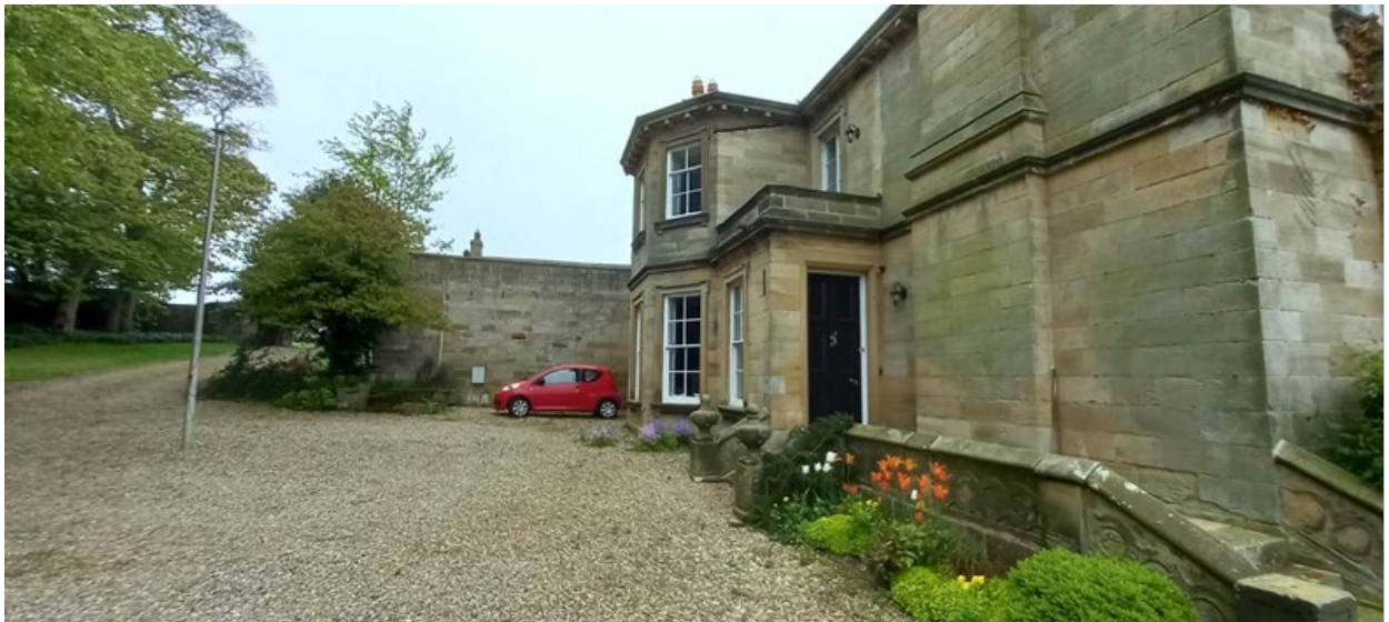
This photograph is taken looking towards the north and the entrance to the dwelling, it shows the west elevation and the proposed location for the orangery and belvedere above the entrance door.
