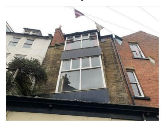
Photograph showing existing New Road elevation of the Dolphin Hotel, Robin Hoods Bay; timber louvre proposed to be installed on existing right hand upper window and metal roof vent to be installed on roof slope.
