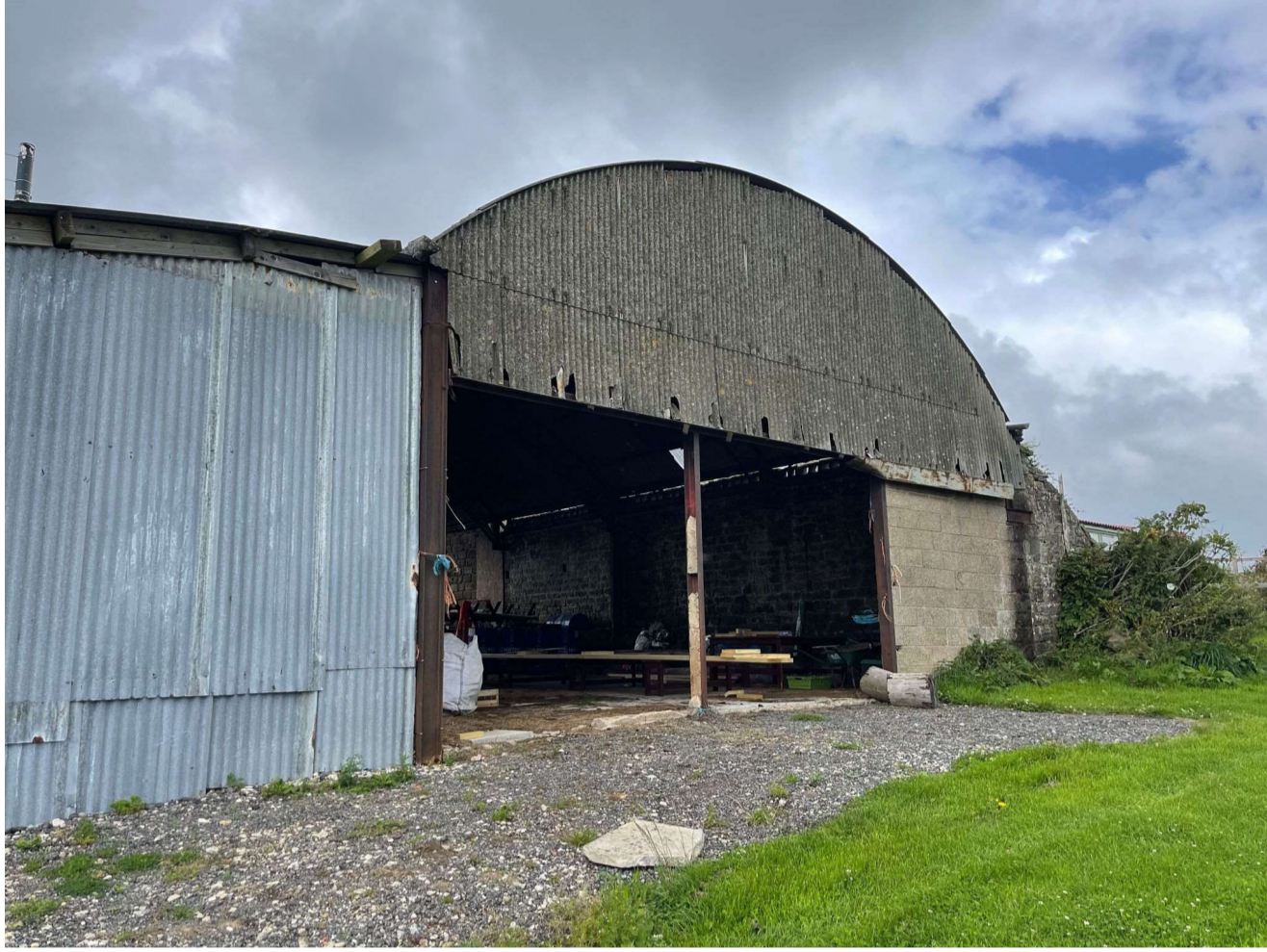
fire damage photo 1
