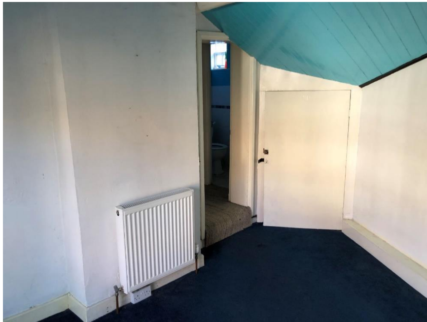
Photo 13 Tapered Room with sloping roof detail
