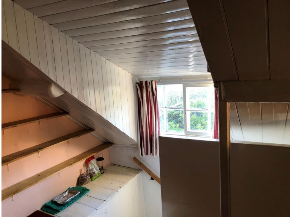
Photo 13 Rear dormer and South East End
