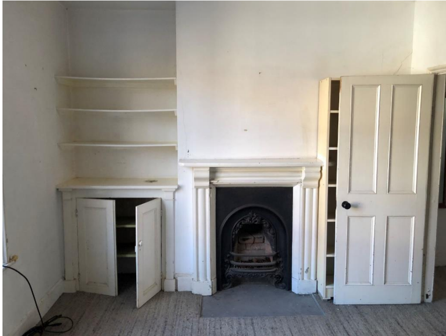
Photo 12 Chimney wall to bedroom
