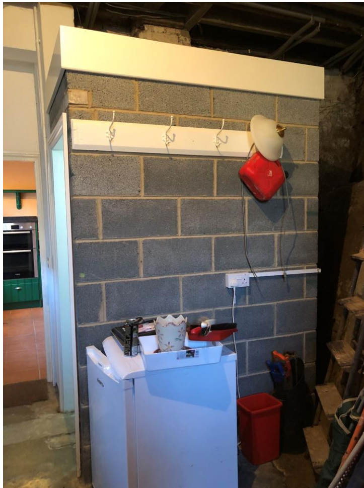
Photo 4 Block WC cubicle, rock face behind in Tapered room
