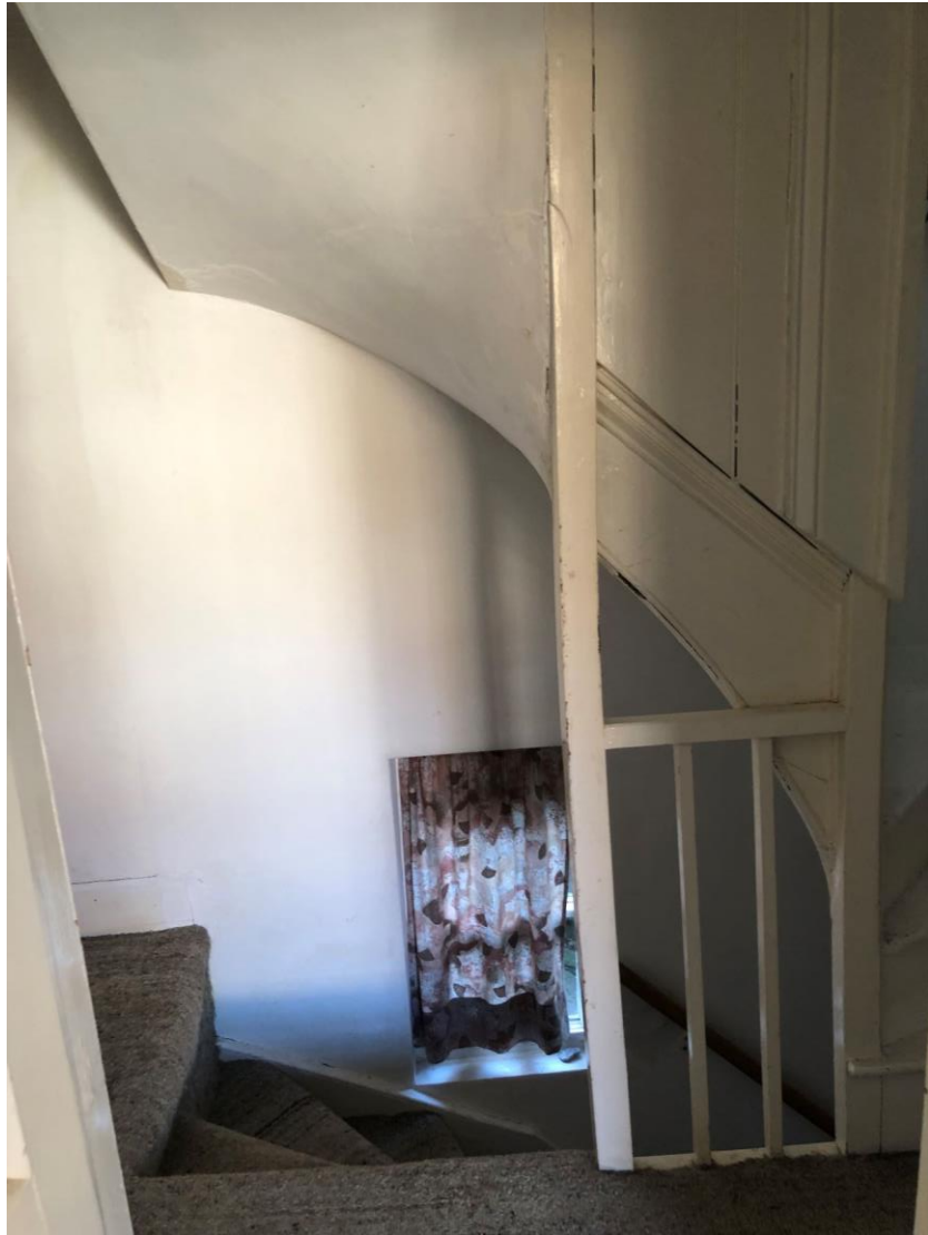
Photo 11 Landing with stair up to Roof space
