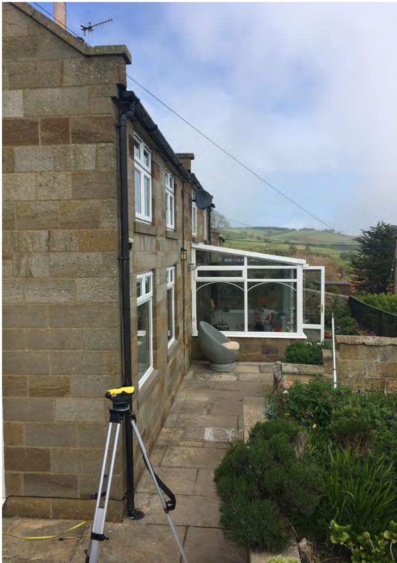
Fig. 19: View looking north east along the south east elevation (front) with uPVC framed conservatory. Contrast with the image in Fig. 33.
