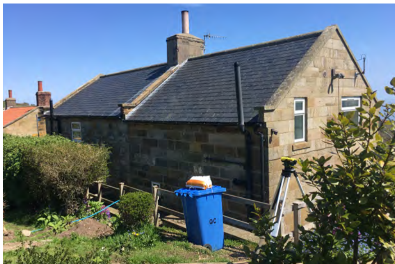
Fig. 25: View looking east to the rear of Quarry Cottage from the parking area, highlighting the significant level change.
