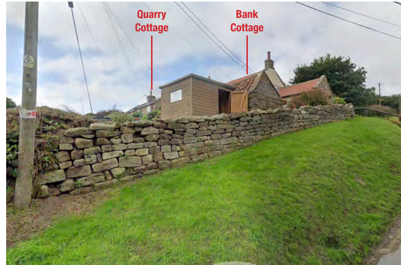
Fig. 6: View looking west from Shop Hill up towards Quarry Cottage on the left and Bank Cottage on the right. Image credit: Google Streetview.
