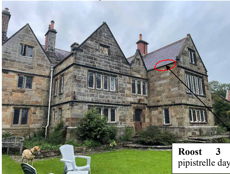
Plate 4 – Thorpe Hall, south elevation
