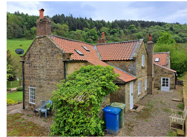
photo of rear elevation and end gable
