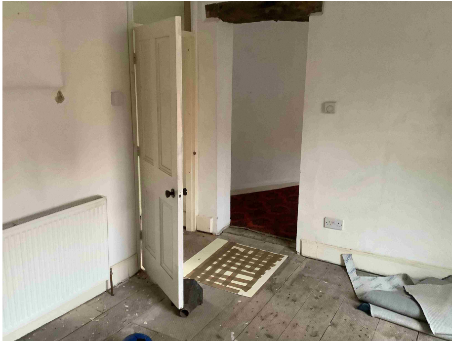
Photo 1 Living room adjacent door to lobby
