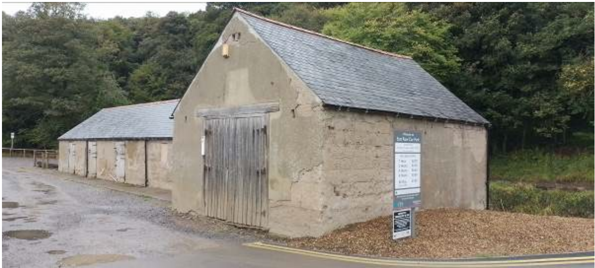
Existing building, located within the pay and display car park in Sandsend
