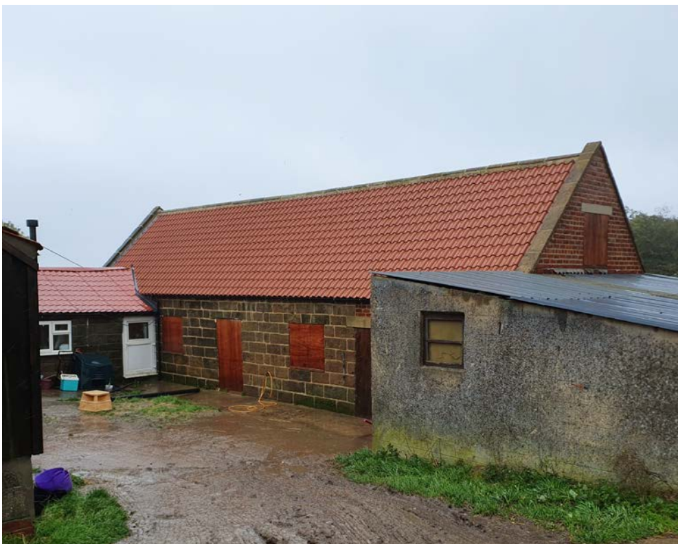
General view of the west and south elevations
