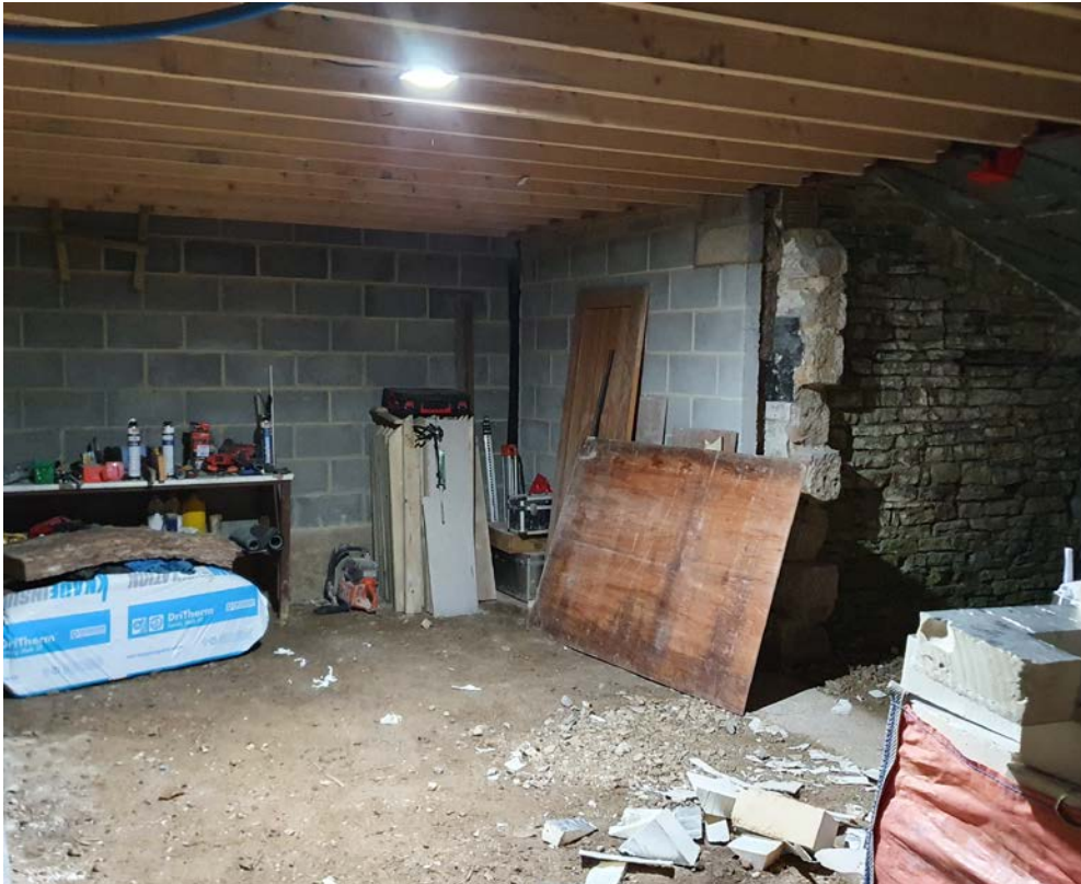
Internal view of the ground floor main room.
