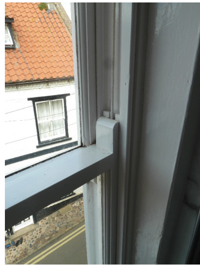
Cracked paint and surface mould indicates general state of decay. Details at sash horn non-vernacular particularly composite planted sections to sash cord channel. These details also apply to W1.
