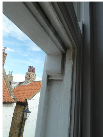
Cracked paint and surface mould indicates general state of decay. Details at sash horn non-vernacular particularly composite planted sections to sash cord channel. These details also apply to W1.
