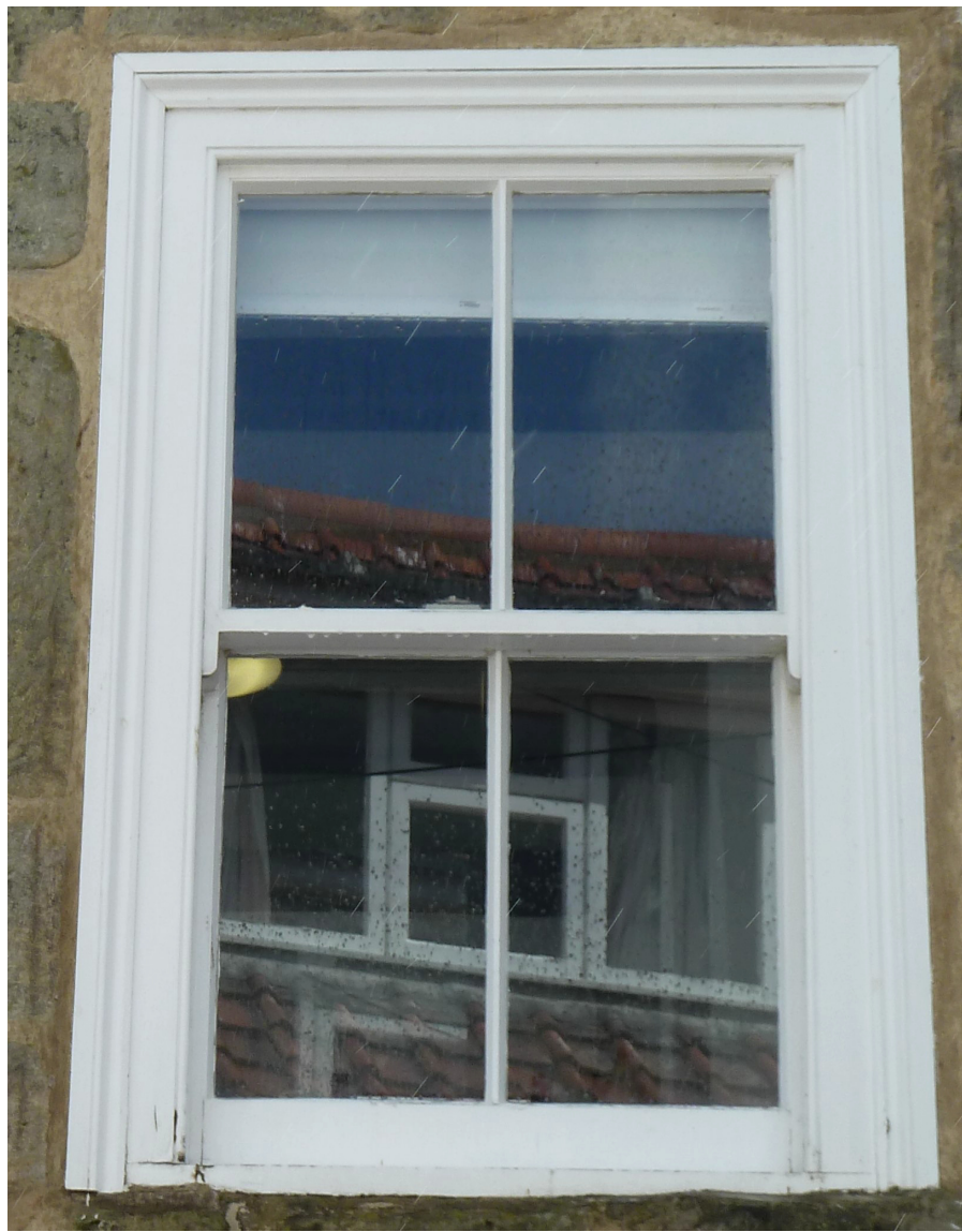
FIRST FLOOR LEVEL BATHROOM. (RHS Viewed Externally).
