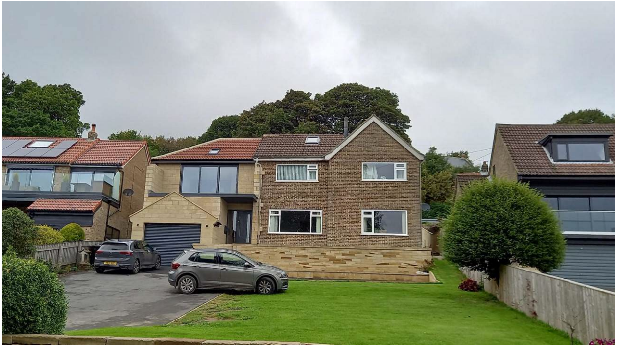
This photograph shows the front elevation of 22 Egton Road, Aislaby.
