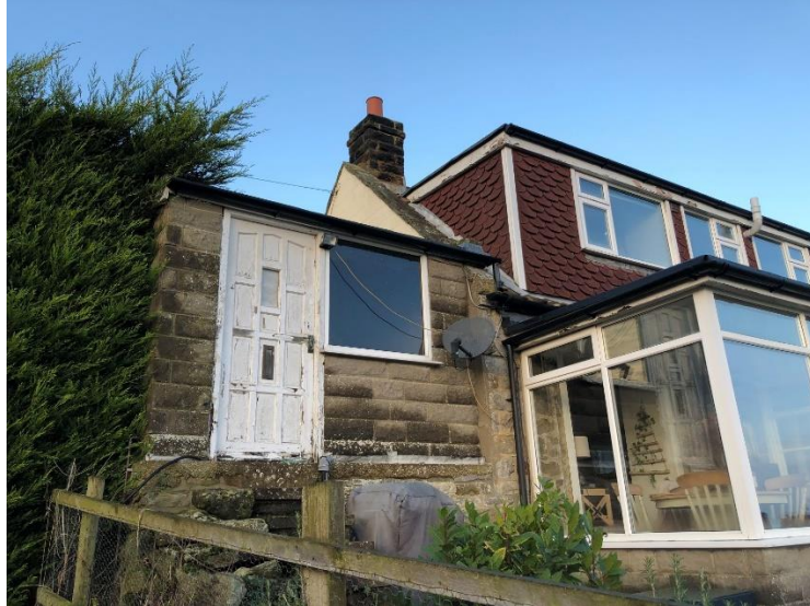
Photo 1 View of part rear elevation
