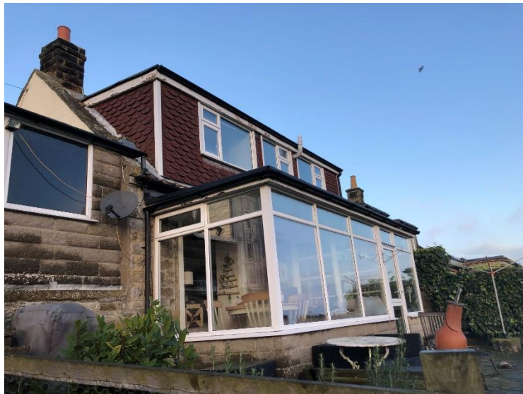
Photo 2 View of part rear elevation 2
