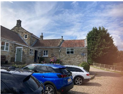
Fig 3 – West facing elevation of Underhill Cottage.
