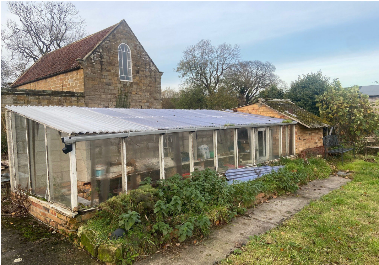
View of the existing greenhouse within the grounds of Thorpe Hall, Fylingthorpe
