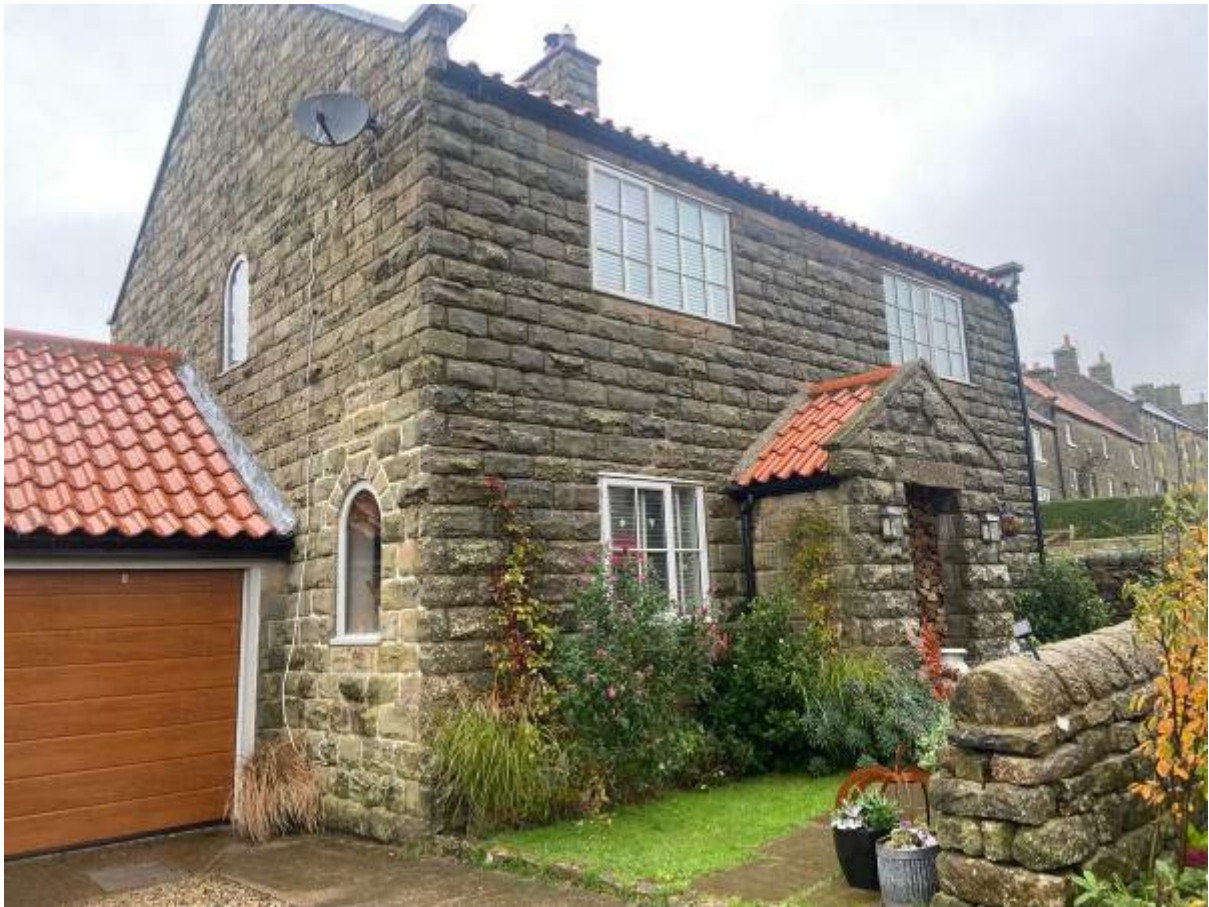
Front and Rear Elevation of Millstones, Egton
